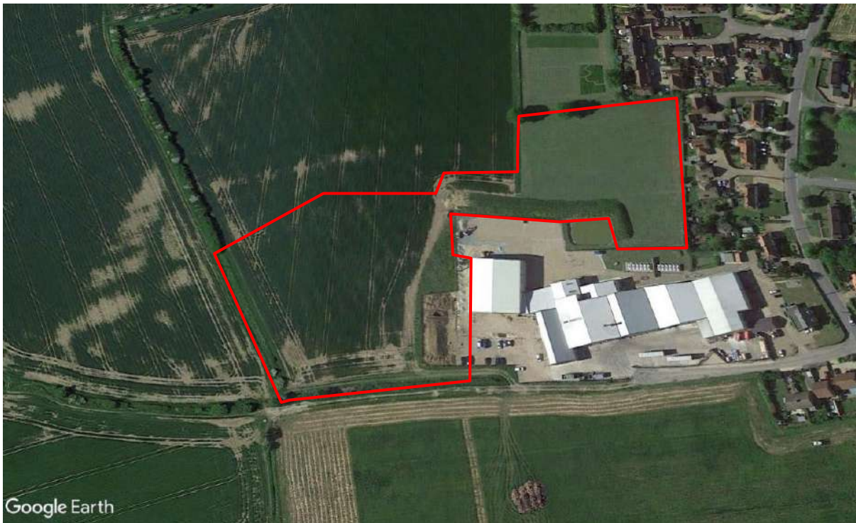
Fig 1: Aerial plan, with approximate site boundary outlined in red. Aerial photograph sourced from Google Earth Pro
