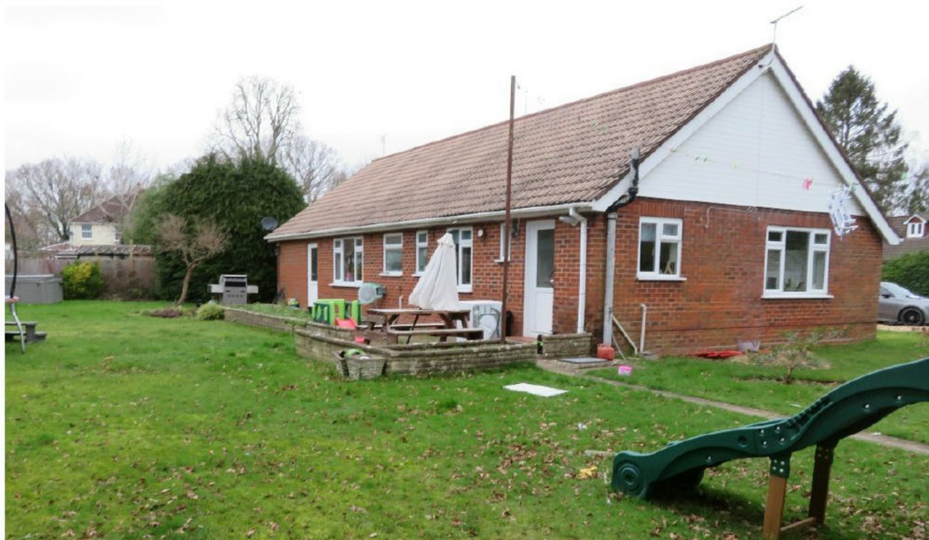
Photo viewing Rear / Side of Property from Back Garden (Camera Facing North)
