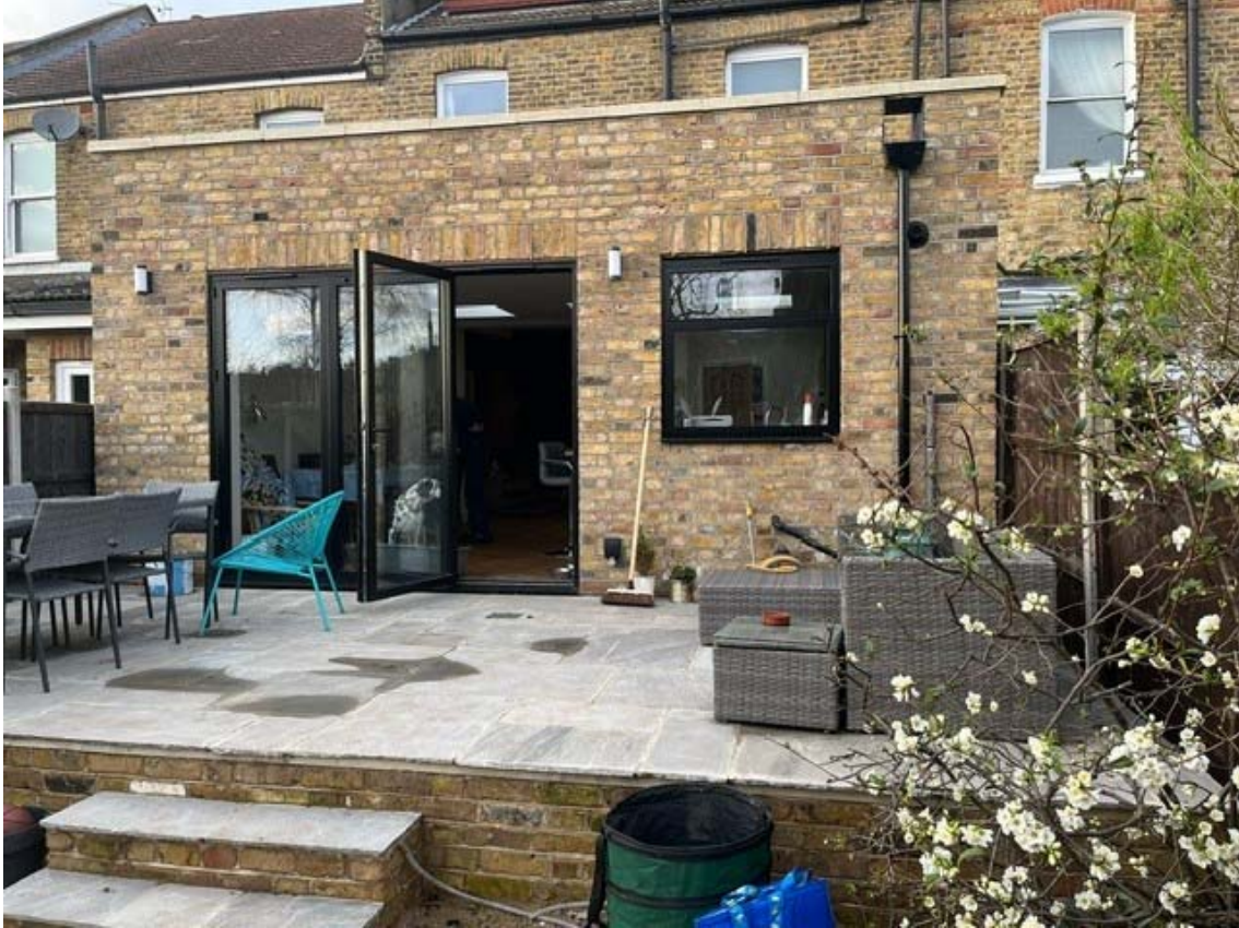
P02- New Rear Extension of No.72 Earlshall Road
