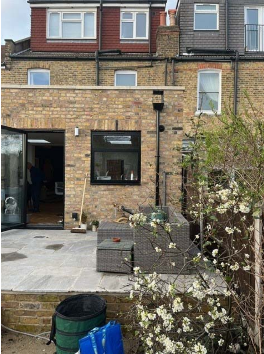
P03- No.72 Earlshall Road and Part of No. 74 Earlshall Road
