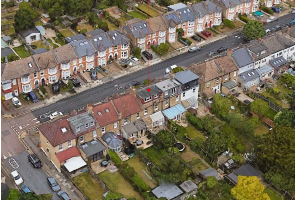
P01- Aerial View of No.72 Earlshall Road
