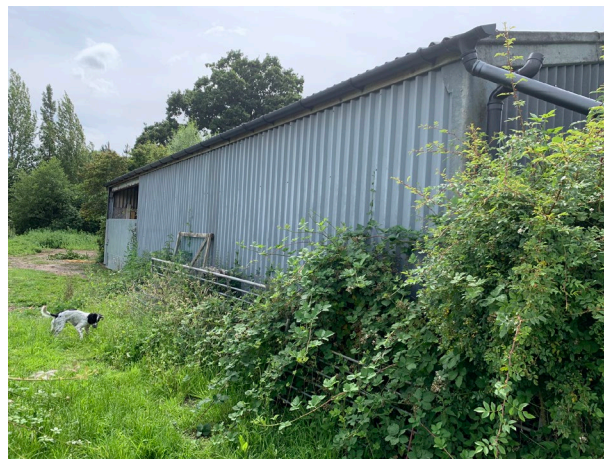
Figure 5 - Photograph of eastern elevation
