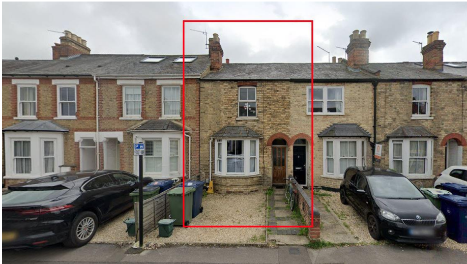
Existing front elevation of 19 Percy St (Google Street View)
