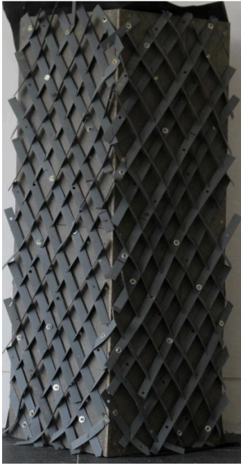
Termination strips on Cement Particle board
