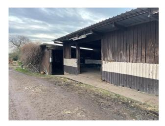
2.2. The Southeast Gable elevation contains an opening to the adjacent field. The remainder of the gable is in corrugated iron sheeting with high level timber boarding. All structural elements are working satisfactorily.
