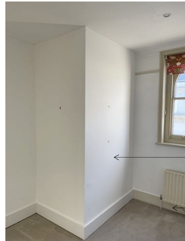
Image 5: Junction of front elevation and non-original partition.
