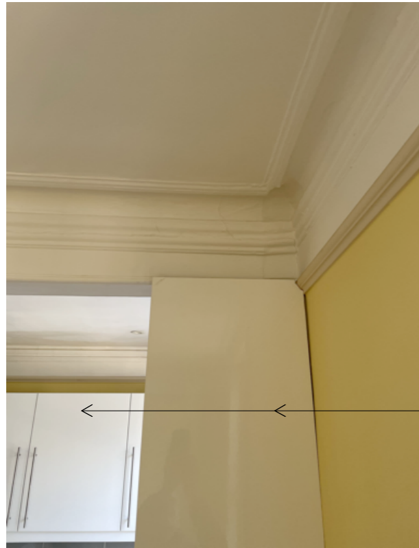
Image 1: Junction between kitchen and rear living room with historic cornice and beam above.
