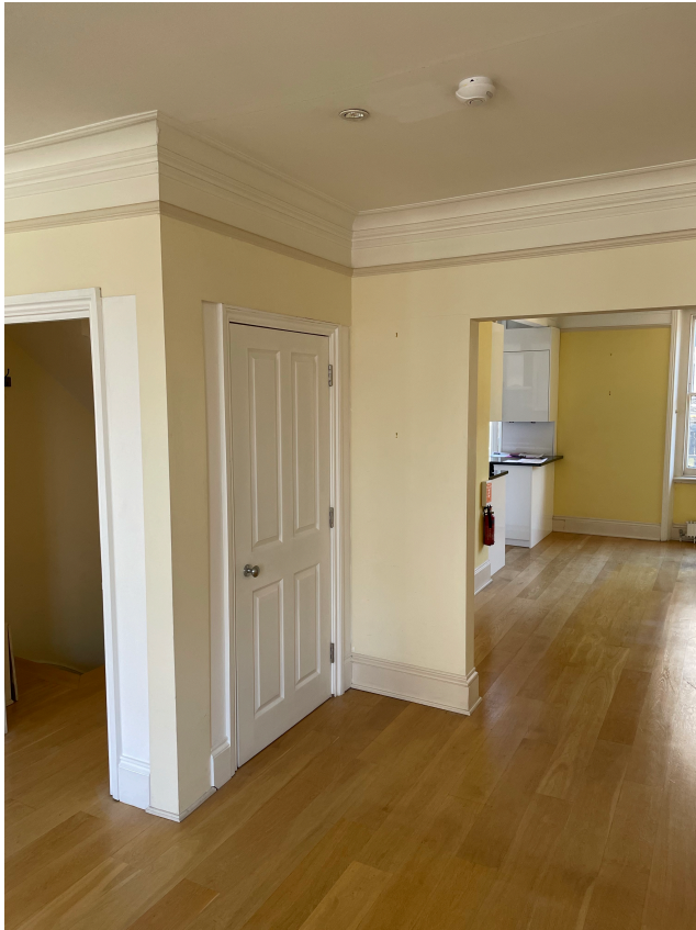
Fig. 1: Existing Condition - 3rd Floor
