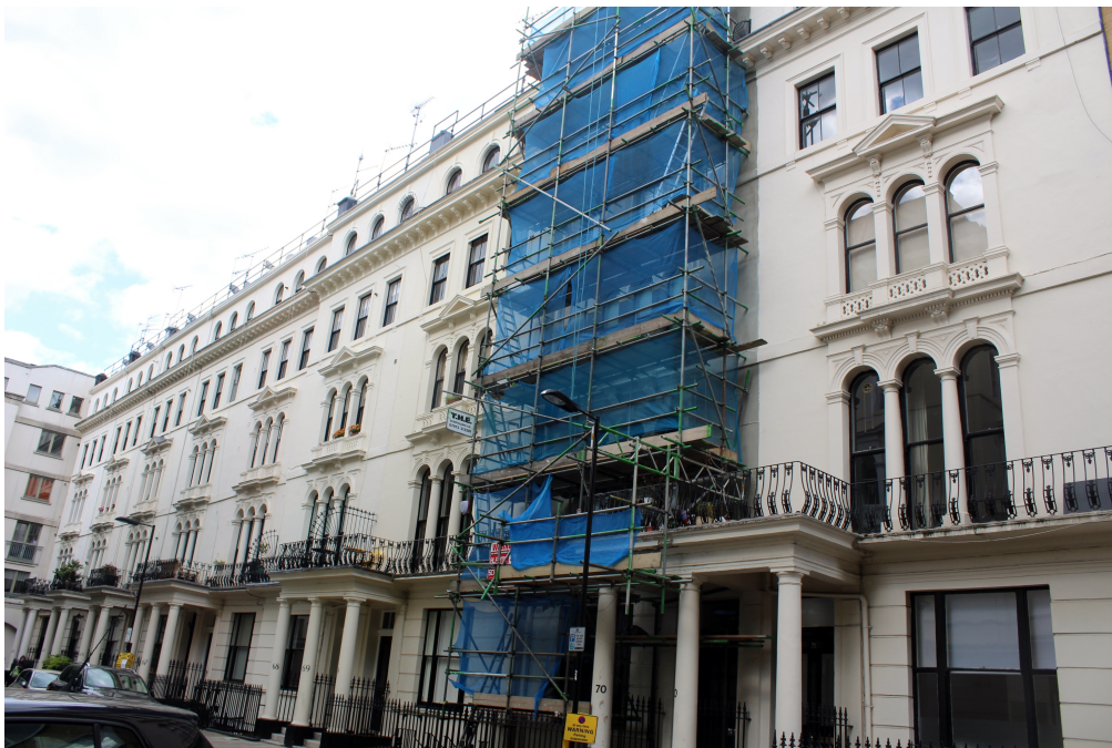
Fig. 1: Front facade of 63-71 Kensington Gardens Square.
