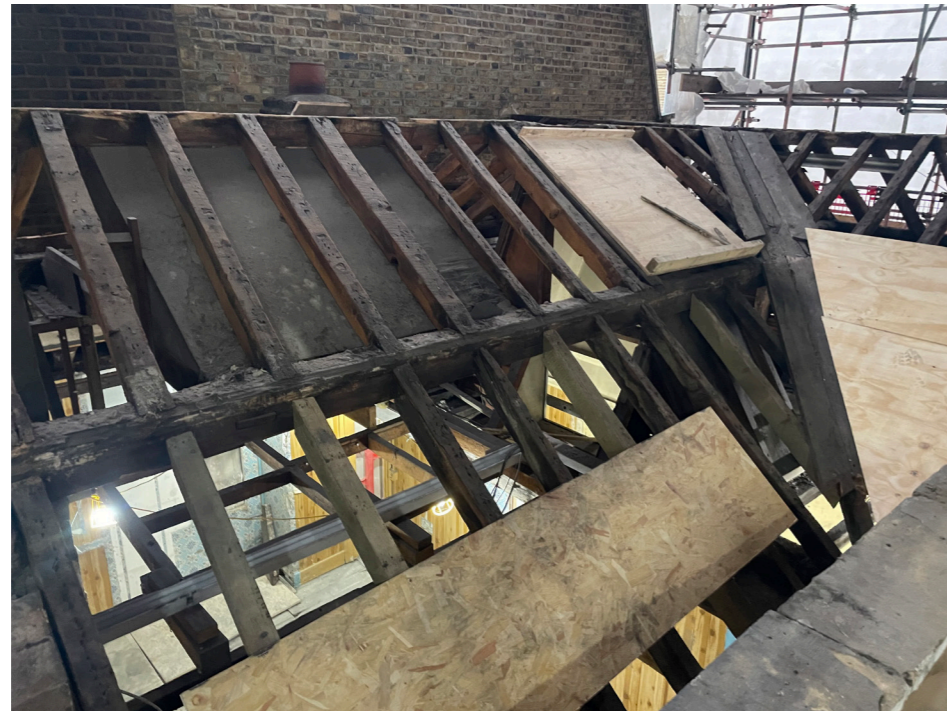
Historic rafters previously replaced, mainly to lower rafters in roof 6
