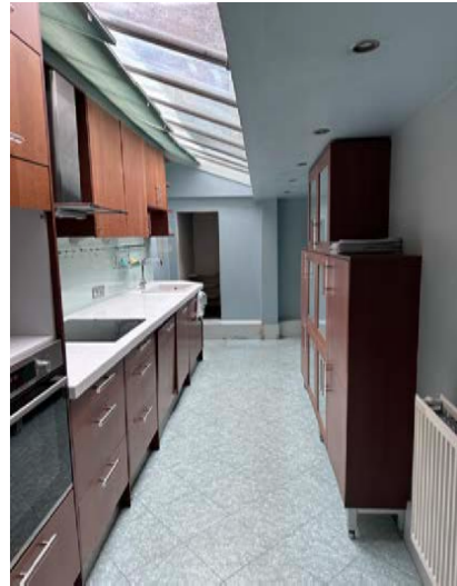
Removal of non original kitchen and masonry spine wall
