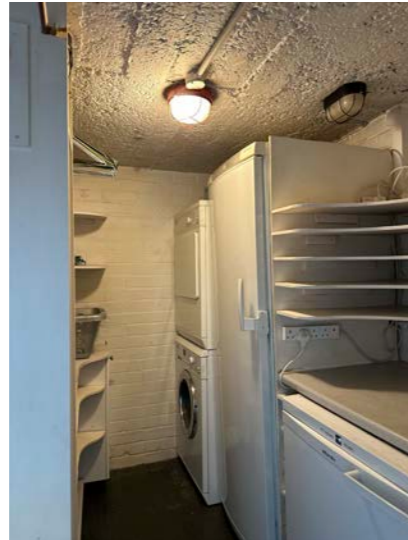
Removal of non original masonry walls and appliances
