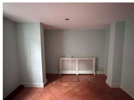
Lower Front Room - removal of masonry nib walls
