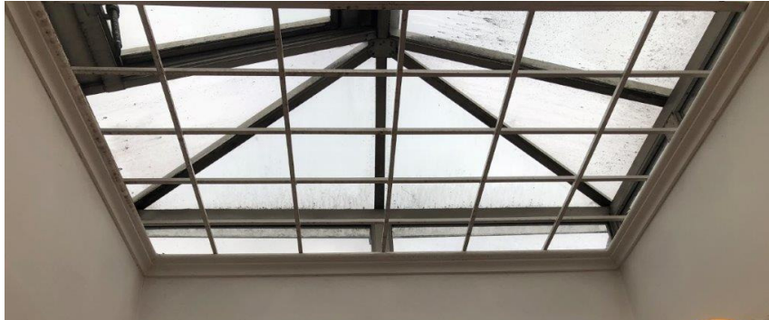
The existing skylight seen from inside Flat 8.
