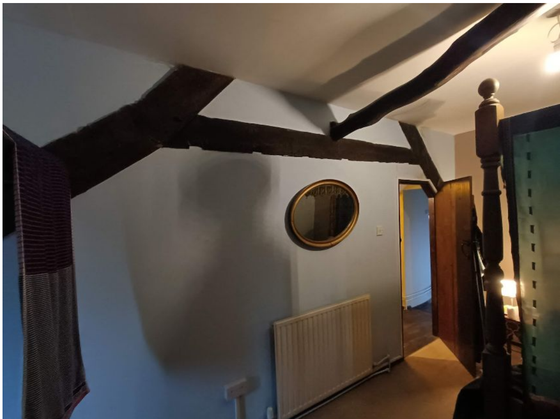
Photo 43: Bedroom 2 showing historic truss
