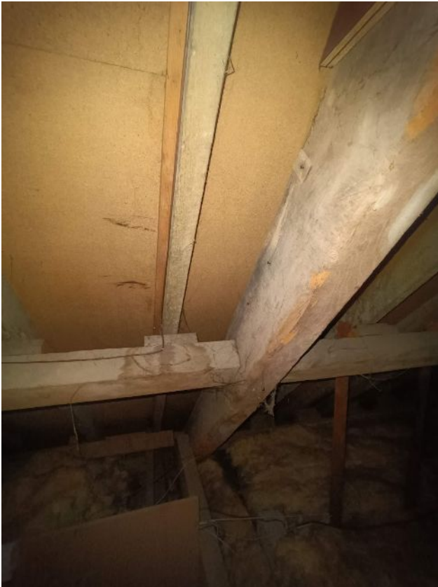
Photo 54: Existing roof construction showing modern elements
