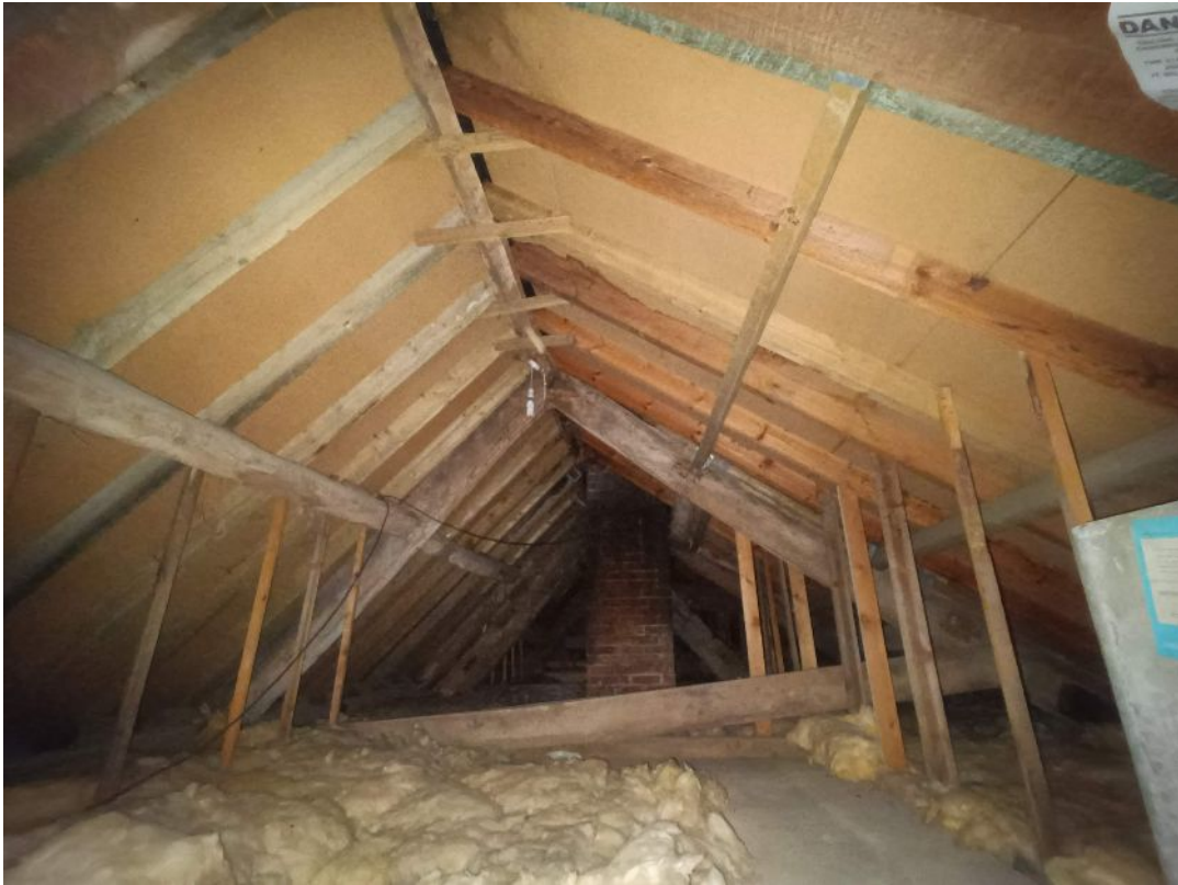
Photo 52: Roof space looking North West
