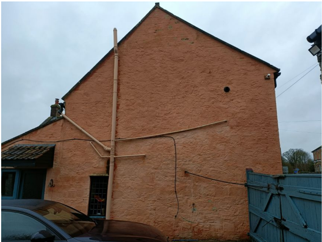
Photo 4: South East Elevation
