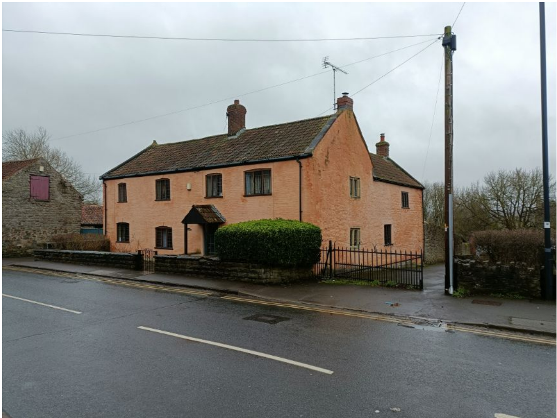
Photo 2: View From North
