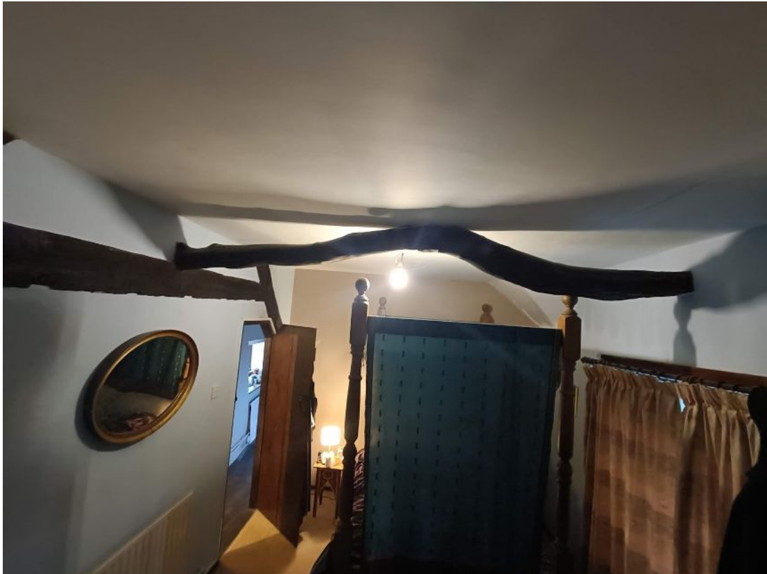
Photo 42: Bedroom 2 Showing historic purlins
