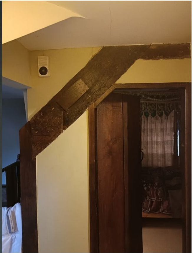
Photo 39: Visible historic rafter - Landing
