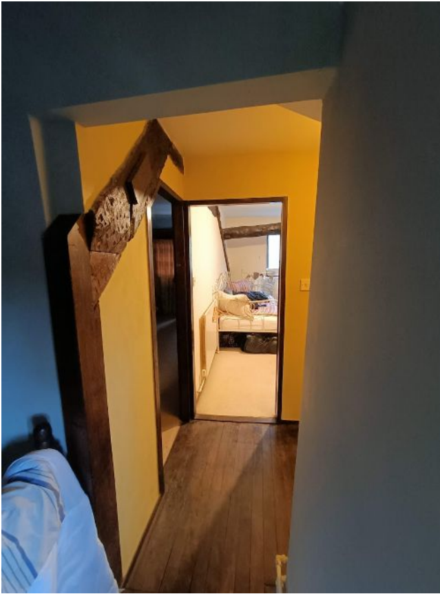
Photo 38: Visible historic rafter - Landing
