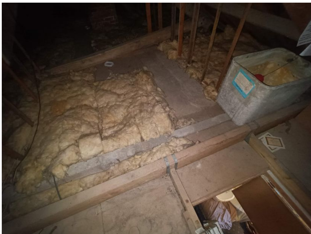
Image 9: View of internal walls from loft showing concrete block construction
