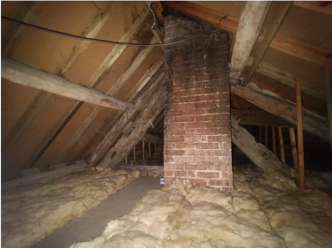
Photo 58: View of main roof showing modern reconstruction and historic elements
