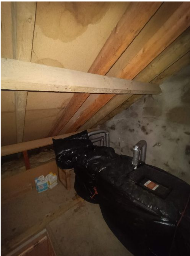
Photo 56: Existing roof construction showing modern elements
