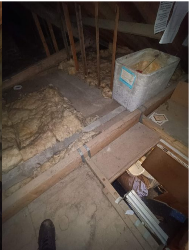
Photo 57: View of top of first floor wall showing blockwork construction
