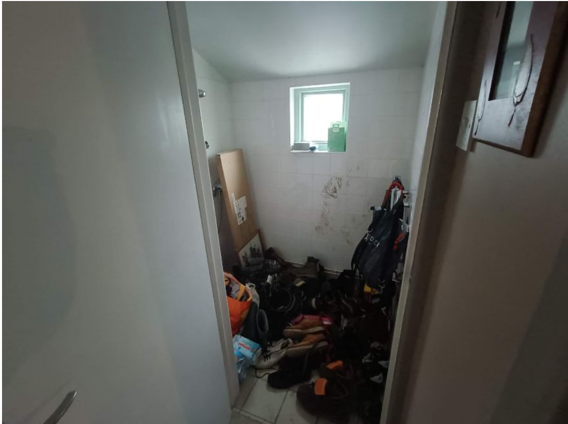
Photo 17: Existing Ground Floor Shower
