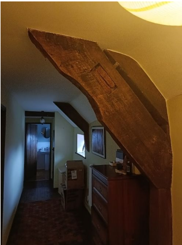
Photo 40: Visible historic rafters - Corridor
