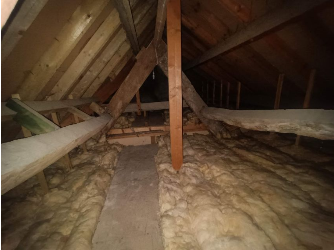
Photo 59: View of main roof showing modern and historic elements
