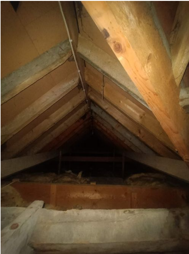
Photo 61: View south west of secondary roof showing modern reconstruction
