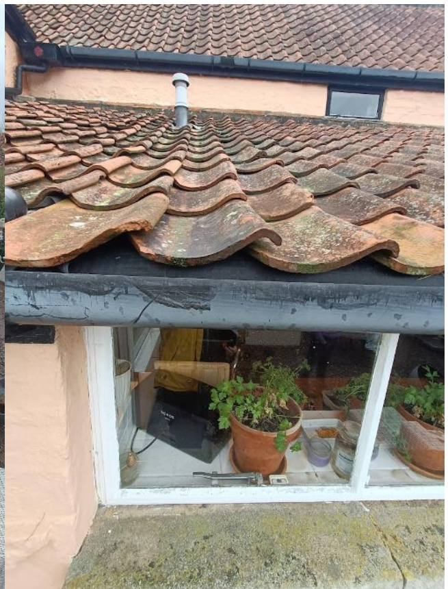
Photo 66: Lean-to roof eaves showing modern vapour barrier
