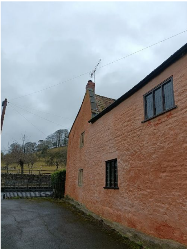
Photo 13: Historic foundations visible NW elevation
