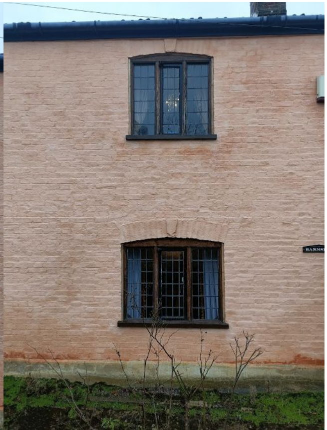
Photo 8: Dining room and Bedroom windows
