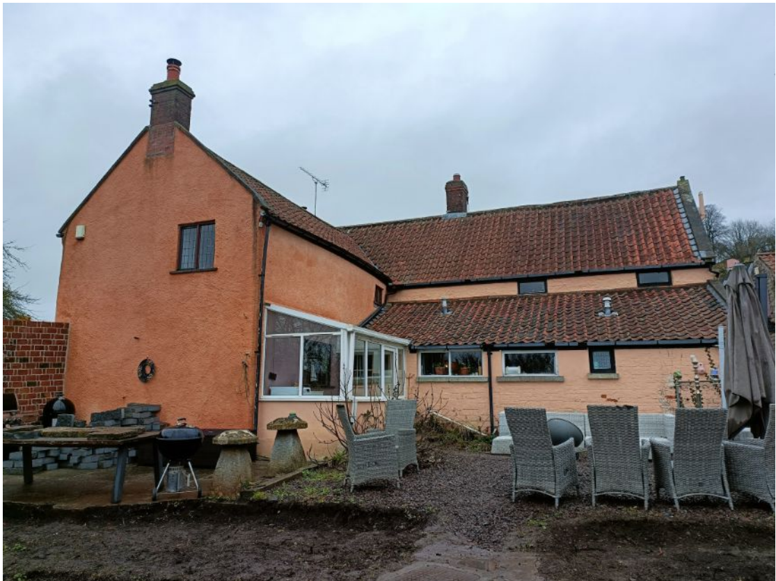
Photo 6: South West Elevation
