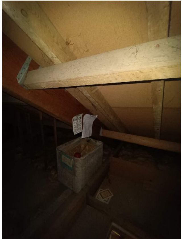
Photo 55: Existing roof construction showing modern elements
