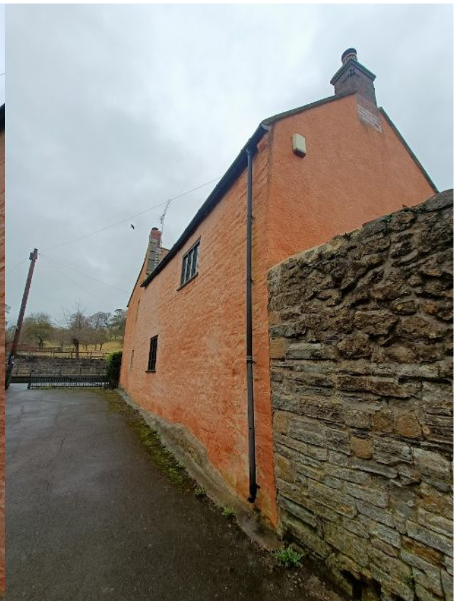
Photo 14: Historic foundations visible NW elevation
