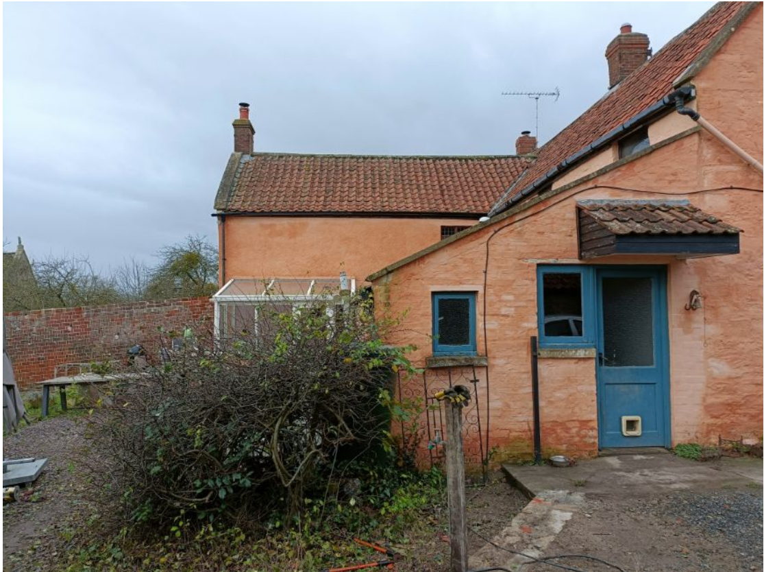
Photo 5: South East Elevation Continued
