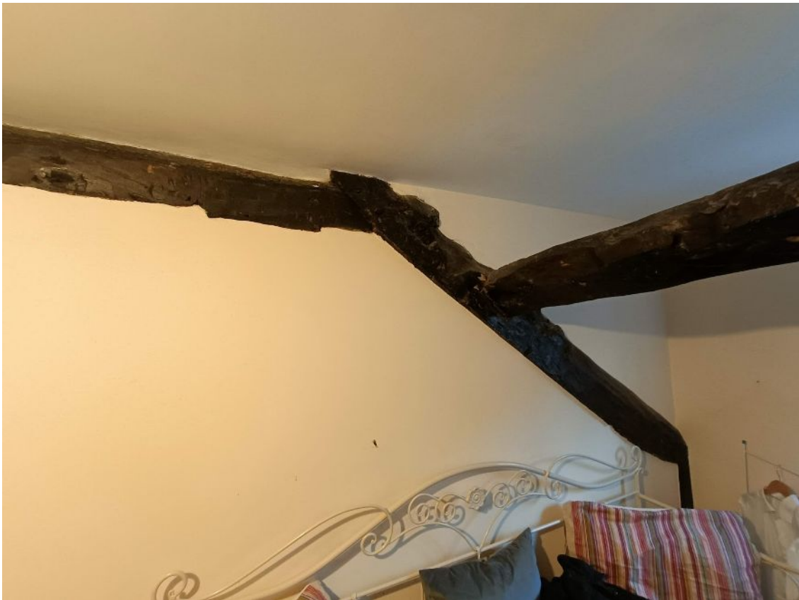
Photo 46: Bedroom 3 showing historic roof elements
