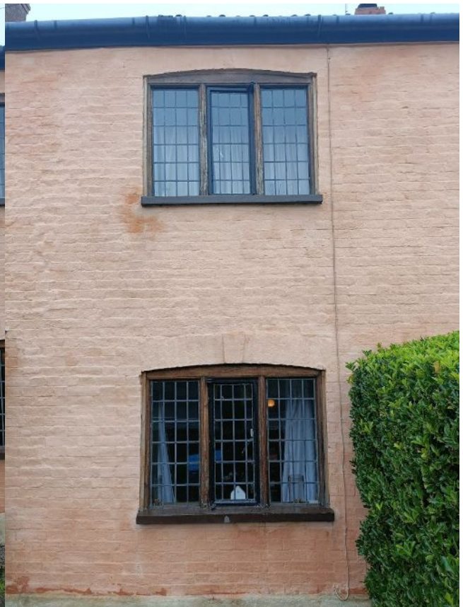
Photo 10: Living room and bedroom windows
