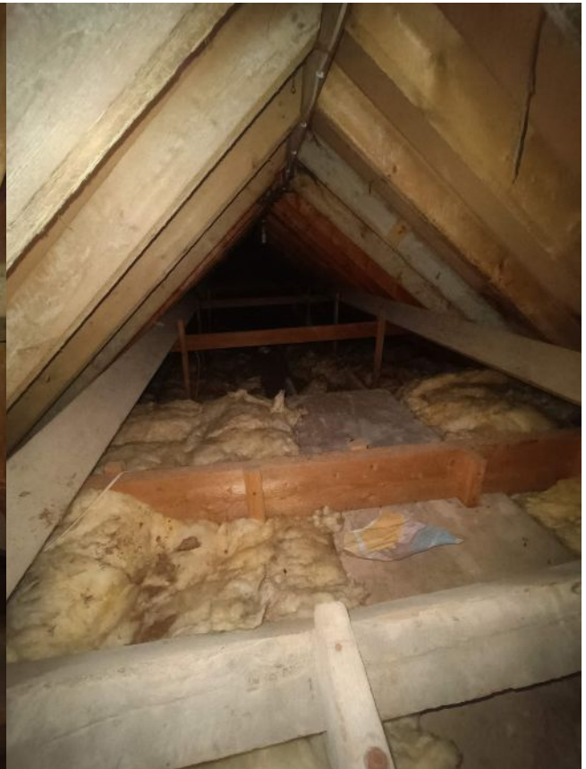
Photo 62: View south west of secondary roof showing modern reconstruction
