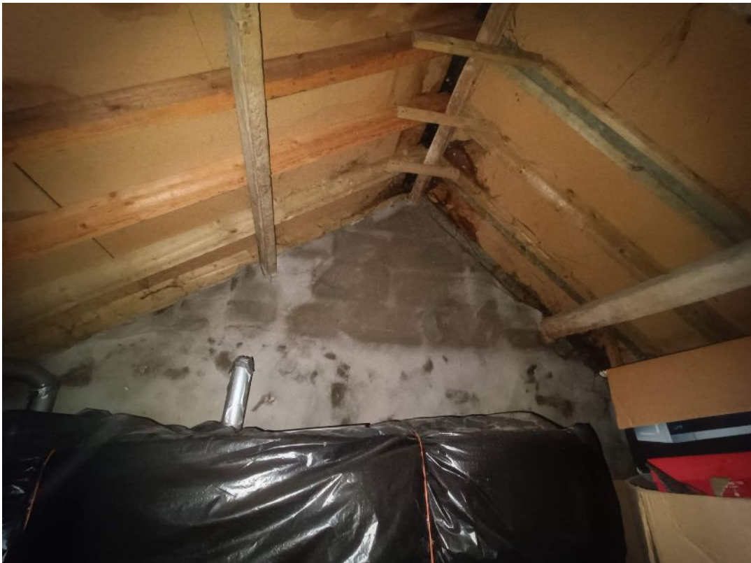
Photo 53: South East gable showing blockwork construction
