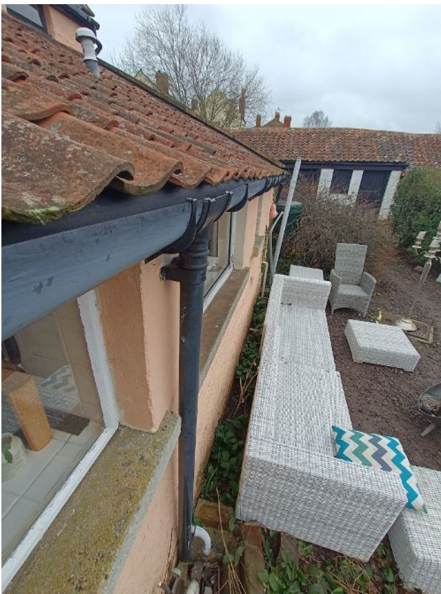
Photo 65: lean-to roof eaves showing modern vapour barrier
