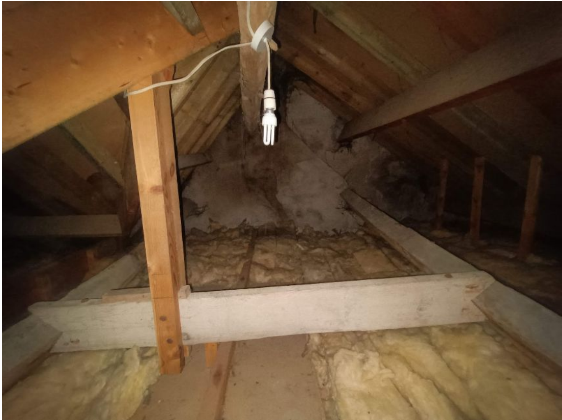
Photo 60: View of North West gable showing original pitch line
