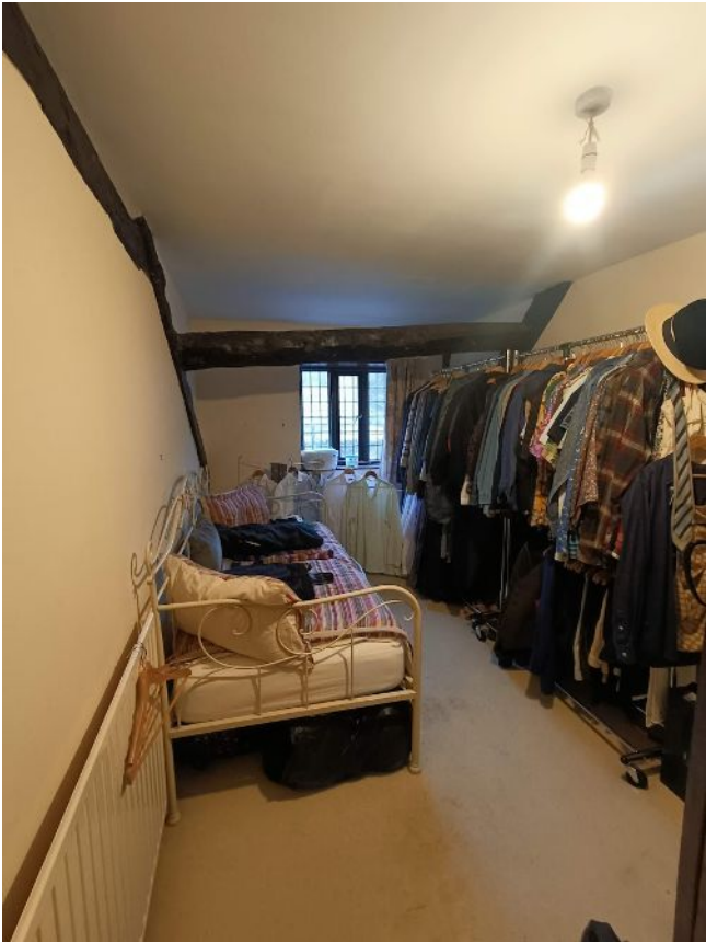
Photo 44: Bedroom 3 showing historic roof elements
