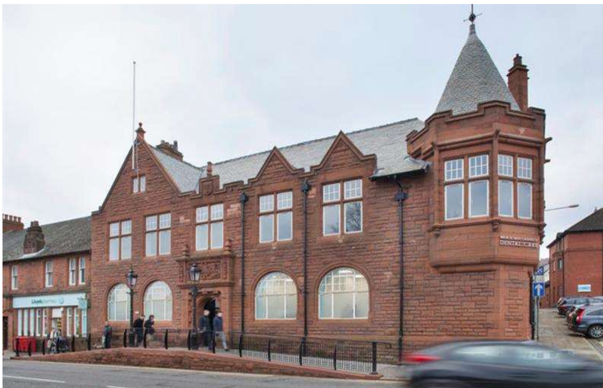
Figure 10: Former Gourock Municipal Buildings: re-slated in Cupa Heavy 3.
