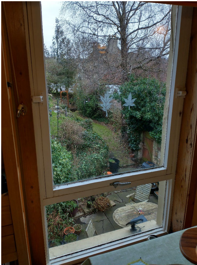
Existing window type – centre hinged
