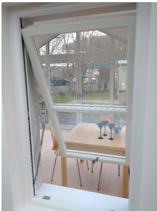
Proposed replacements – white painted hardwood frames, H- fold, 20mm air gap (without centre frame section shown in these photos). They will look identical to the existing windows when closed.
