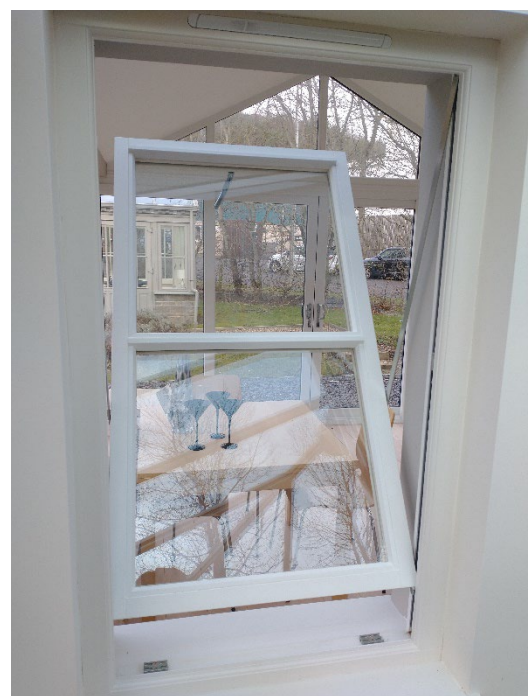
Proposed replacements – white painted hardwood frames, H- fold, 20mm air gap (without centre frame section shown in these photos). They will look identical to the existing windows when closed.
