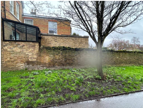
Existing wall images
