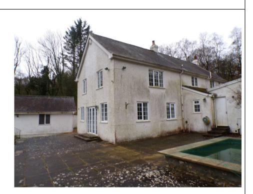
Photo taken of the West side of the dwelling showing the Perspex link roof to be replaced and the position of the proposed porch over the annexe rear door.
