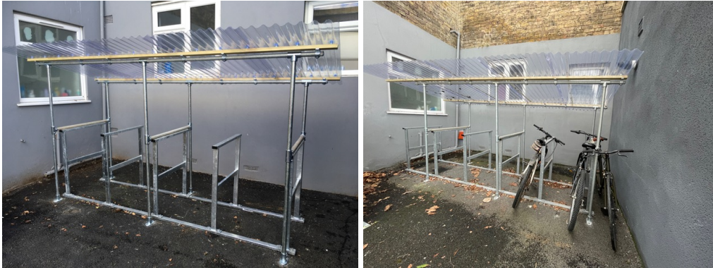
Figure 1 - Cycle store (left) as previously installed for 10 cycle parking spaces, now extended (right) to provide 12 cycle parking spaces (Eco Cycle Shelter Range supplied by Urbanfab Street Products)
