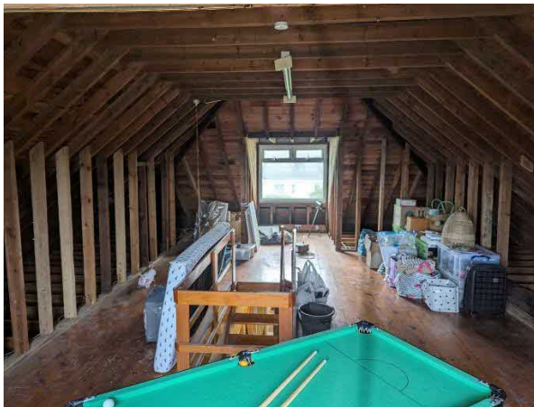
Photo 4. Showing the room in the roof space looking south
