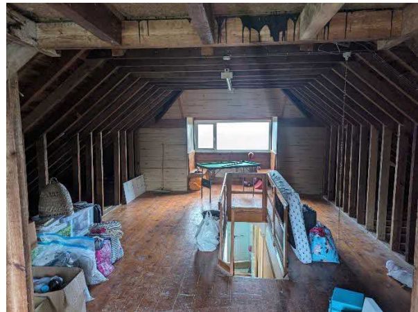
Photo 5. Showing the room in the roof space looking north
