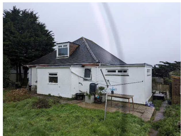
Photo 2. Showing the property from the south east
