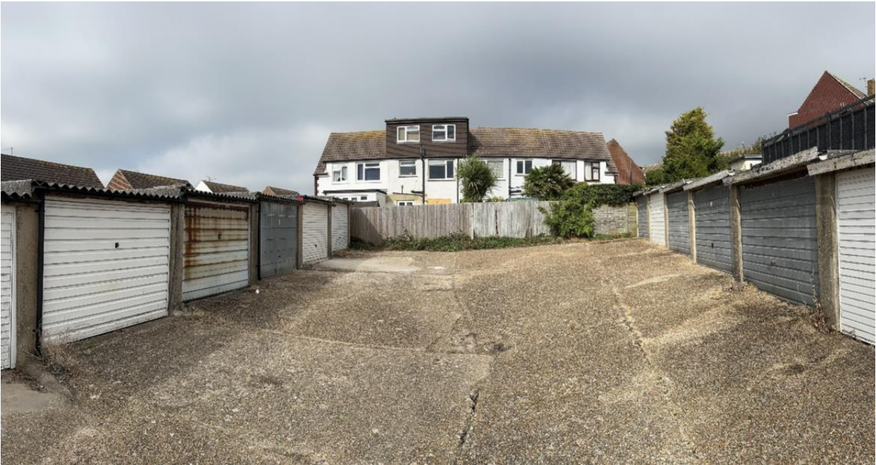
View of site looking towards the North boundary:
