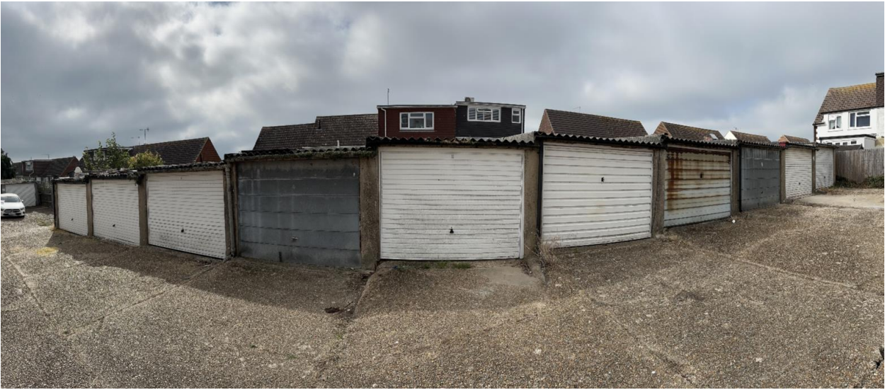
View of the west boundary (rear of houses in Broomfield Drive):
