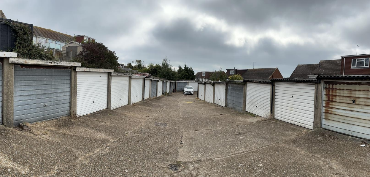
View of the site looking towards the south boundary:
