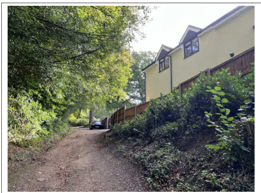
Existing Dwelling adjacent to road
