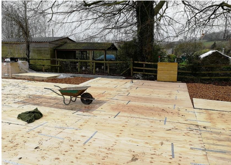
Figure 6 – Plywood sheeting used as ground protection.
