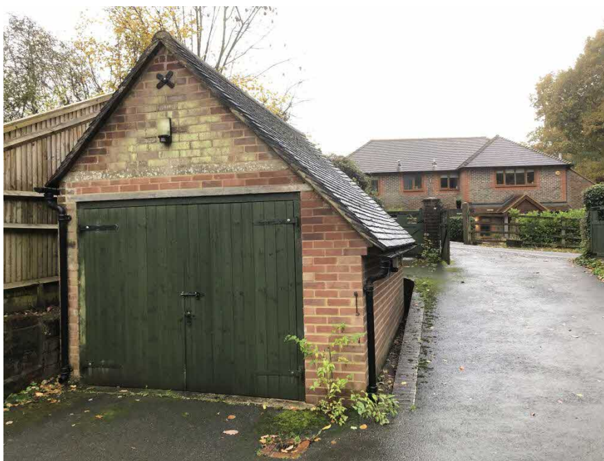
Neighbours Drive & Garage Adjacent
