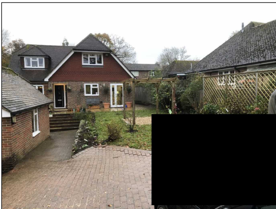
Front Garden View from street – Right Side
