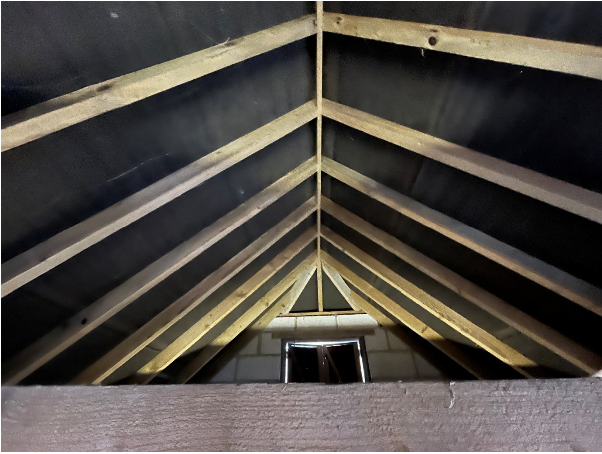
Figure 5. Garage roof looking northeast.
