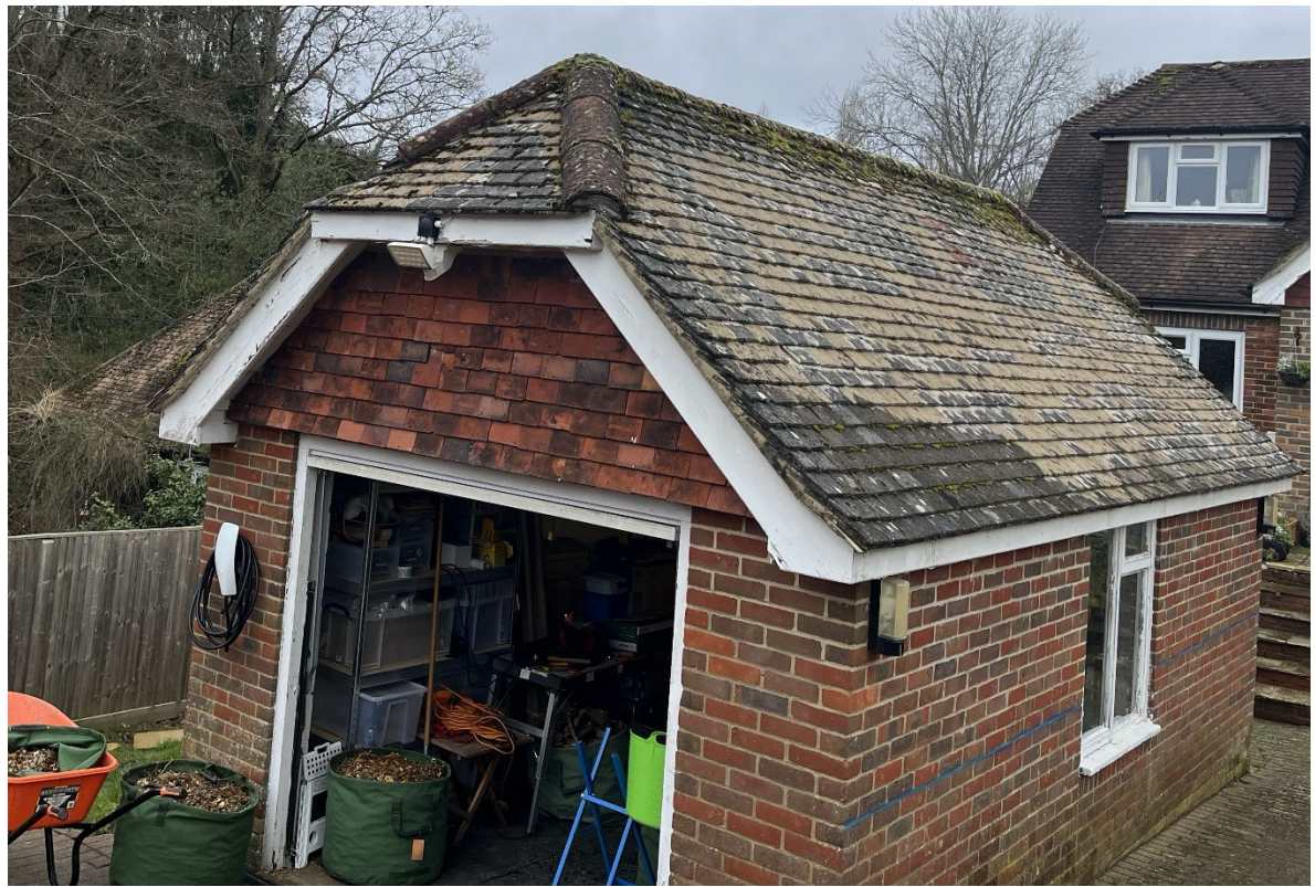
Figure 2. Southern and eastern elevation of garage looking north.
