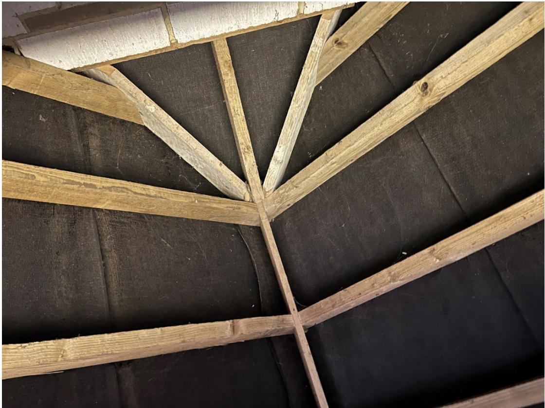
Figure 4. Garage roof looking southwest.
