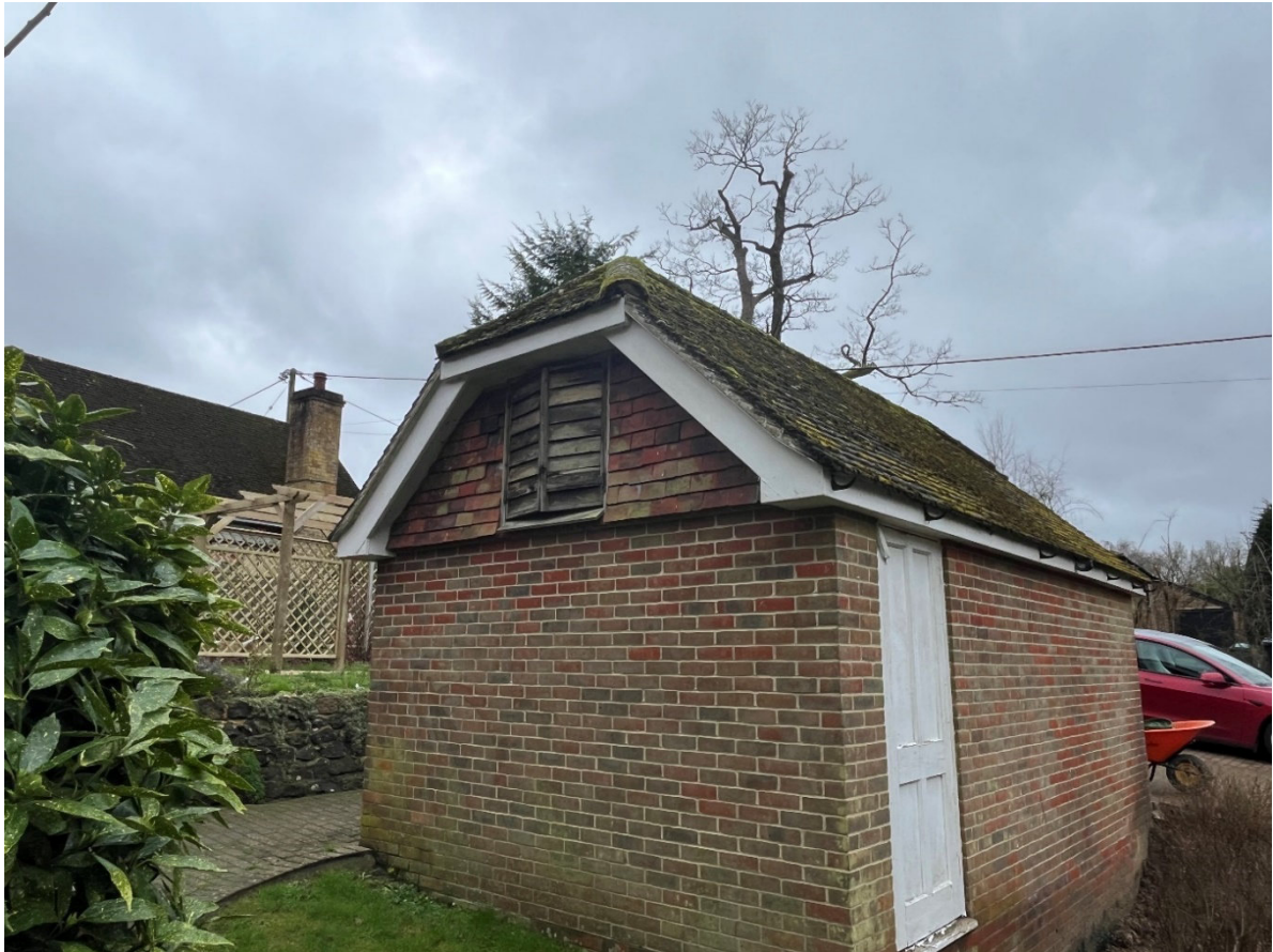
Figure 1. Northern and western elevation of garage looking south.
