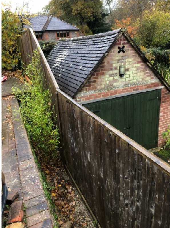
Neighbours Garage –adjacent to proposed Garage location
