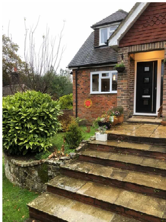
Existing Step access –New Ramp Location
