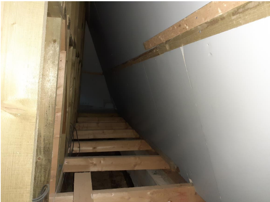
Image 04 – Loft void within the mansard roof of building B1.
