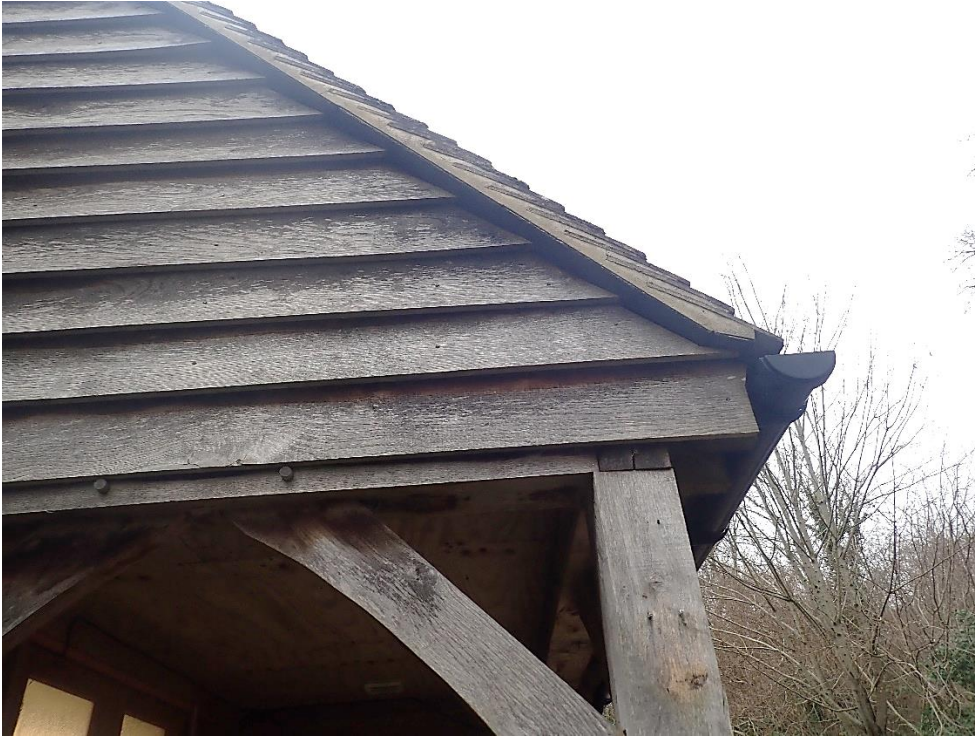
Timber weather-boarding above wood store
