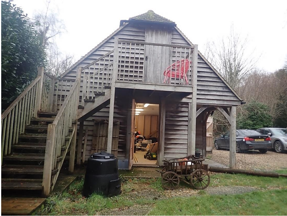
The car barn, viewed from the south
