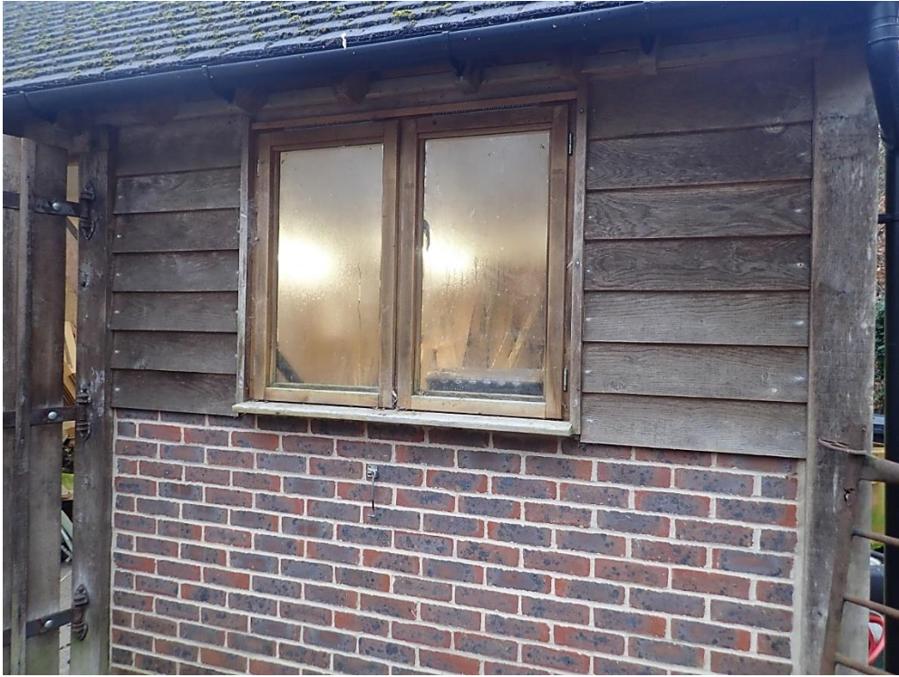
North-east section of car port wall
