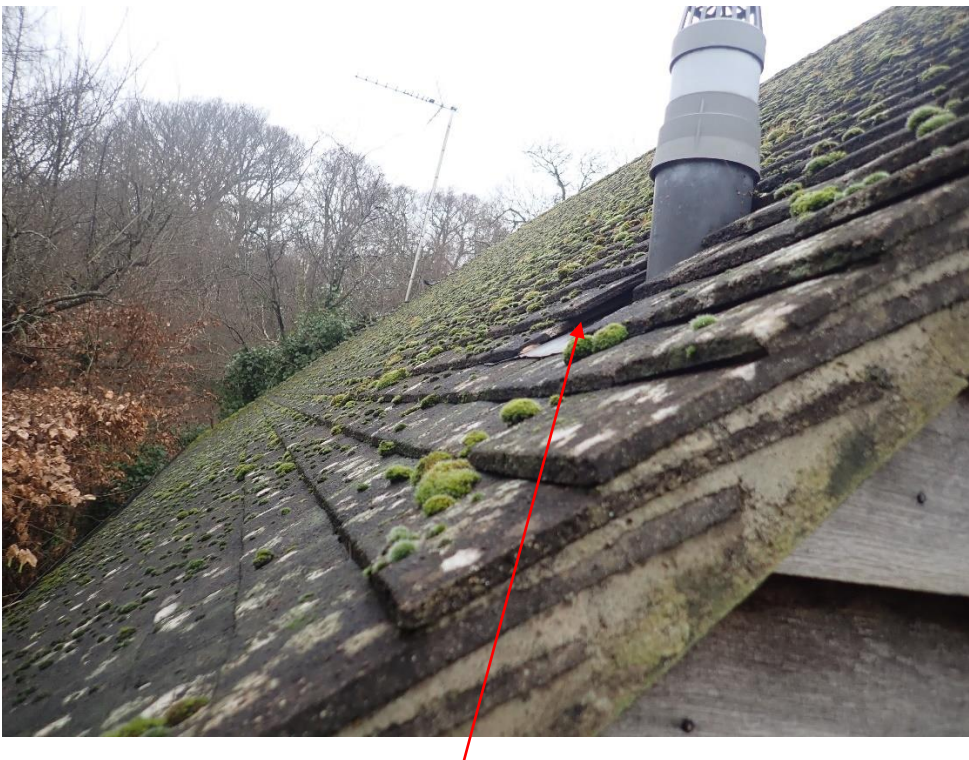
Tight-fitting concrete roof tiles with single small crevice
