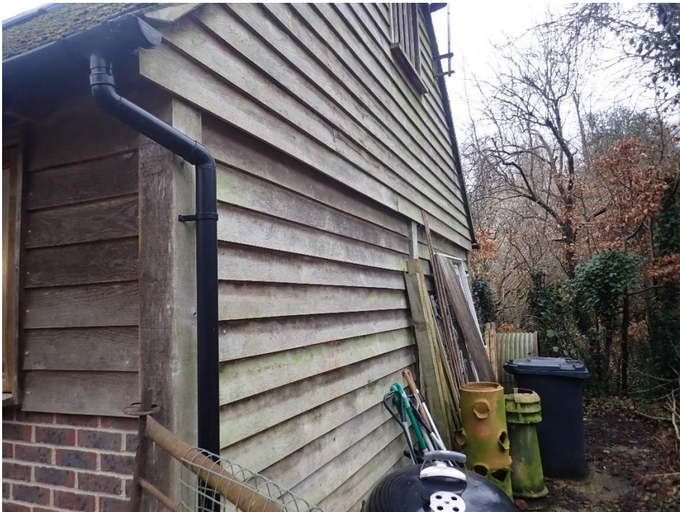
North end wall of car barn
