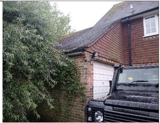
Photograph 4: Western elevation of the extension and partial northern elevation of the house, with tile hangings visible
