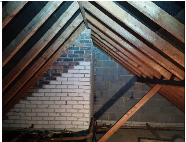
Photograph 2: Roof void above the single-storey extension
