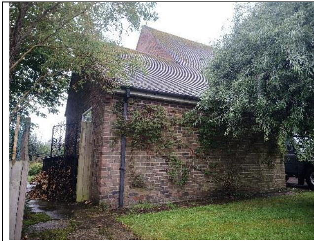
Photograph 3: Northern elevation of the extension
