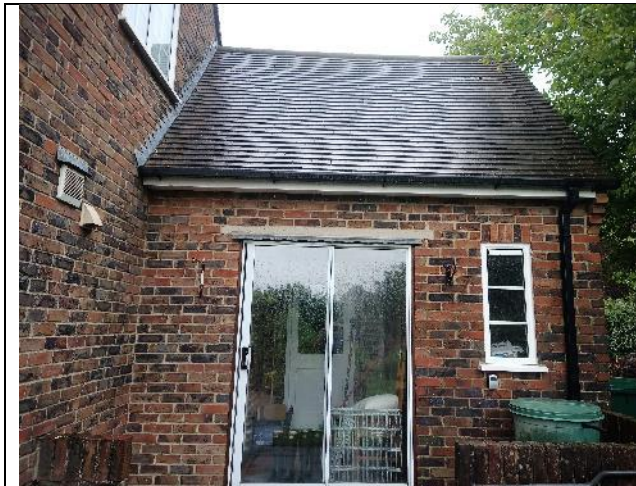
Photograph 1: Southern elevation of the extension and eastern elevation of the house
