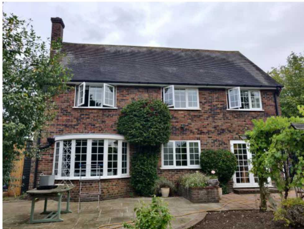
REAR ELEVATION (SOUTH-WEST) VIEWED FROM REAR GARDEN
