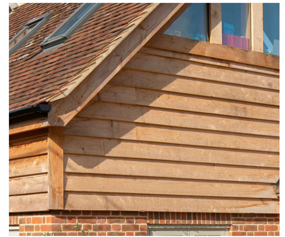
Example of douglas fir cladding
