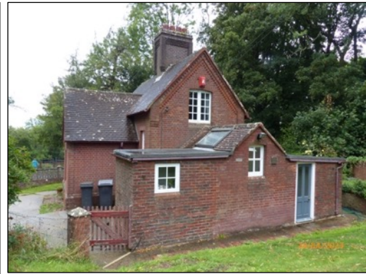
Figure 2: Eastern elevation, showing existing single storey extension.
