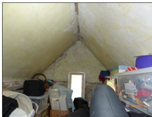
Figure 5: Void 3 – showing plastered ceiling and window at southern end.
