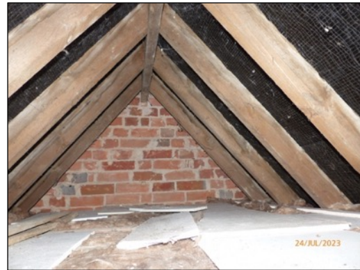
Figure 4: Void 2 – extends in an easterly direction from the central chimney.
