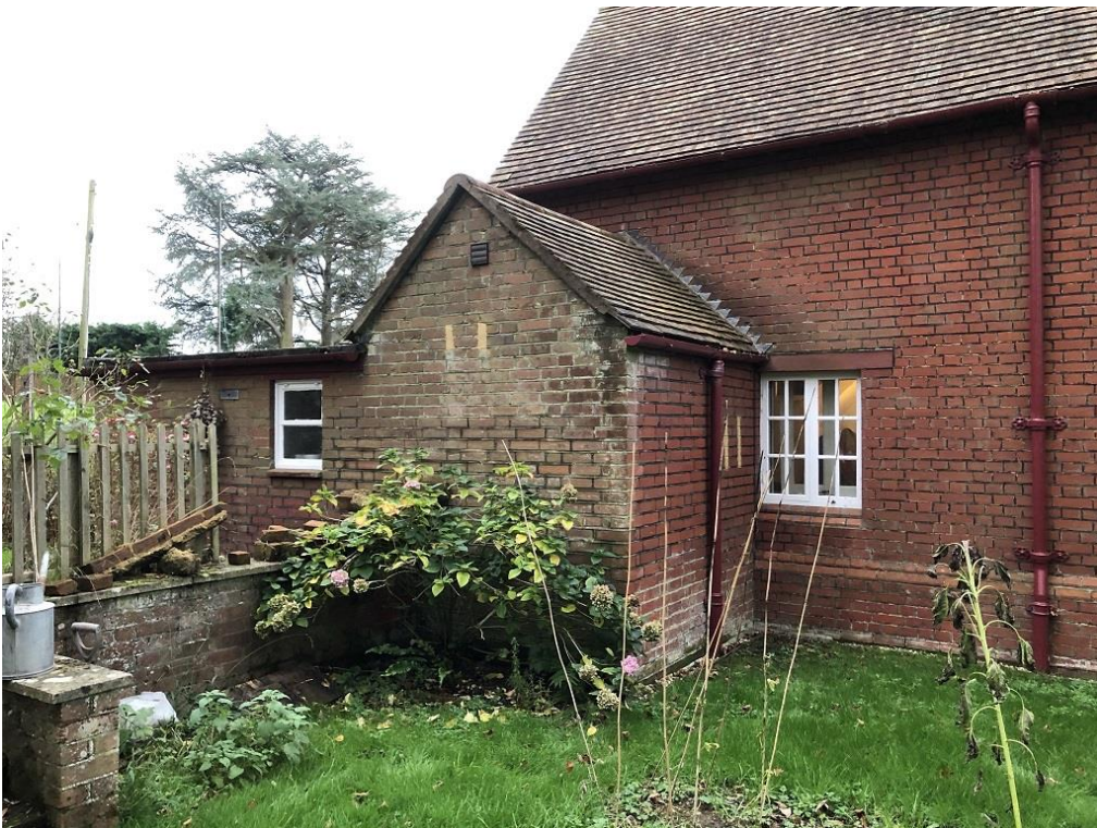
5.08. North elevation 2 looking south.
