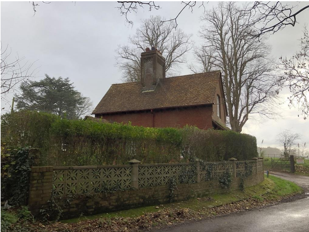
5.12. North elevation looking south from Park Lane.
