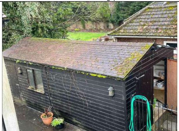
B2 Shed. The building is in an excellent condition with no potential roosting features for bats.
