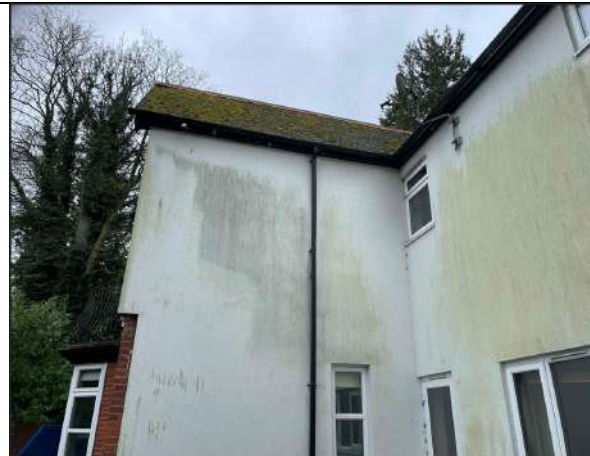
Eastern elevation of B1 Dwelling.
