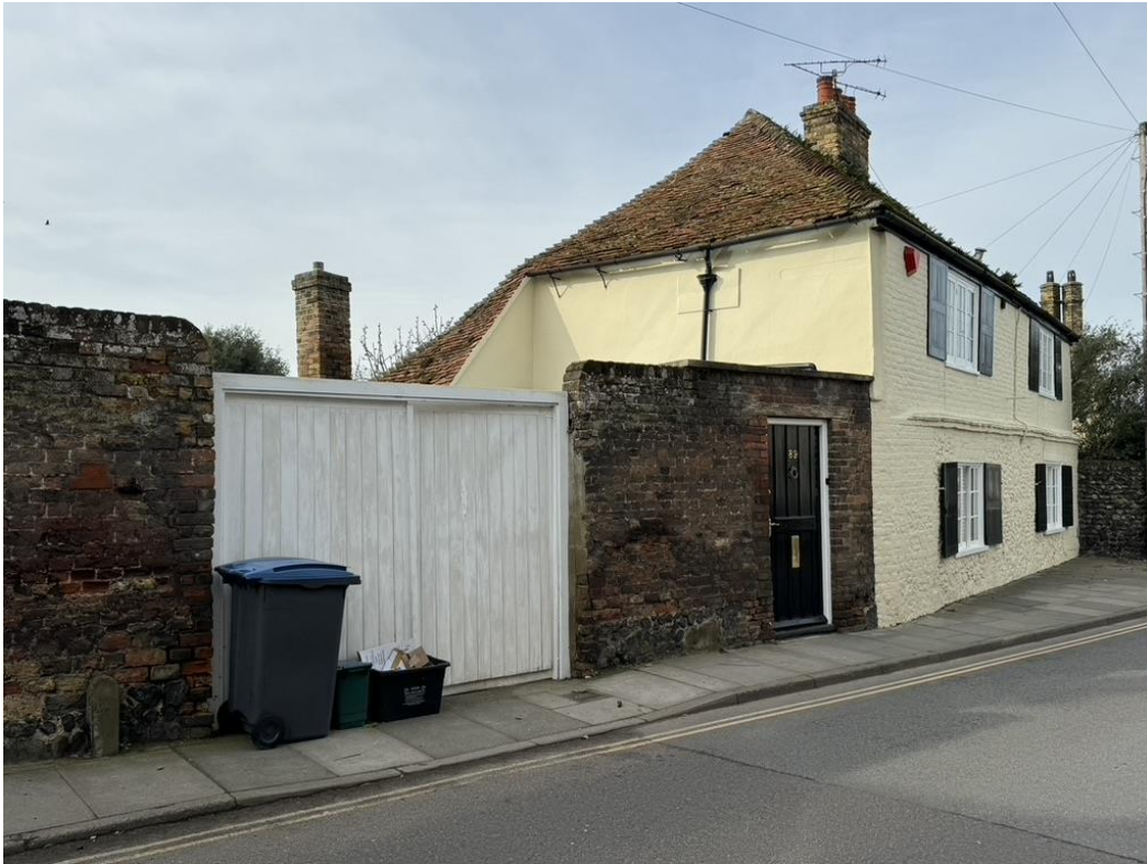
Photo (i) – Existing street elevation showing gates
