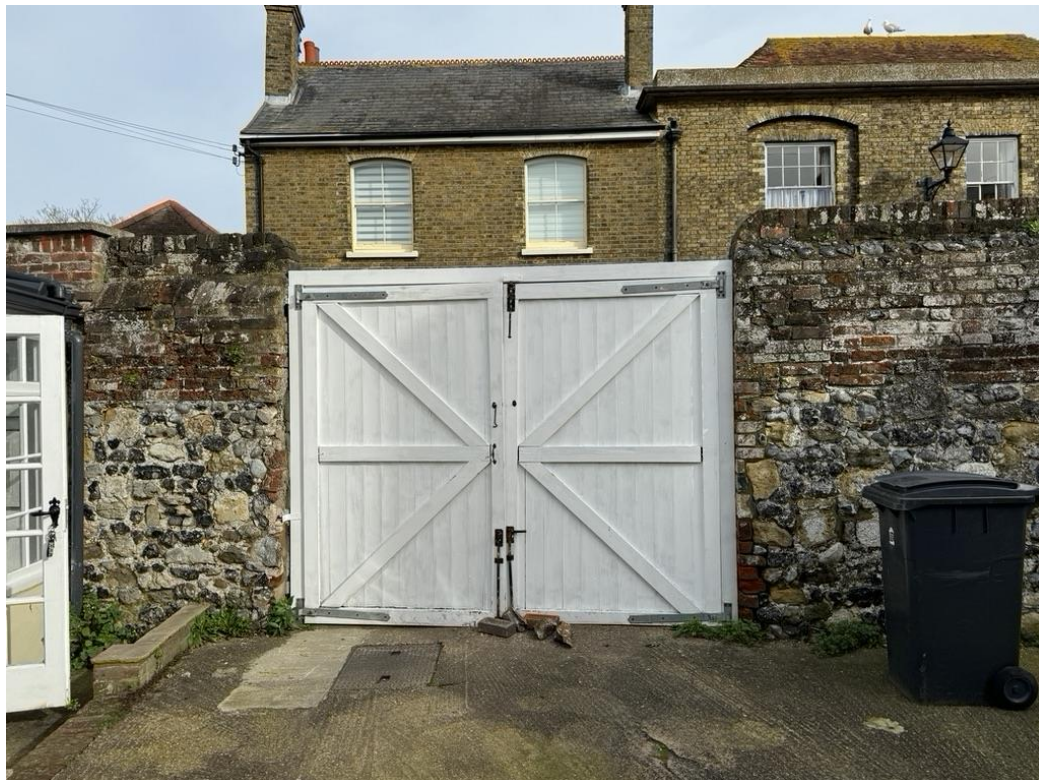
Photo (ii) – view of existing gates inside the courtyard
