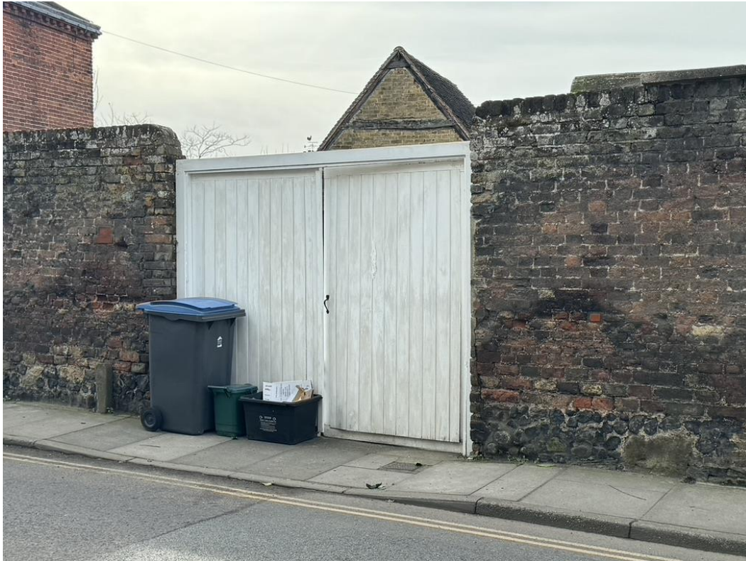
Photo (i) – view of gates from the road
