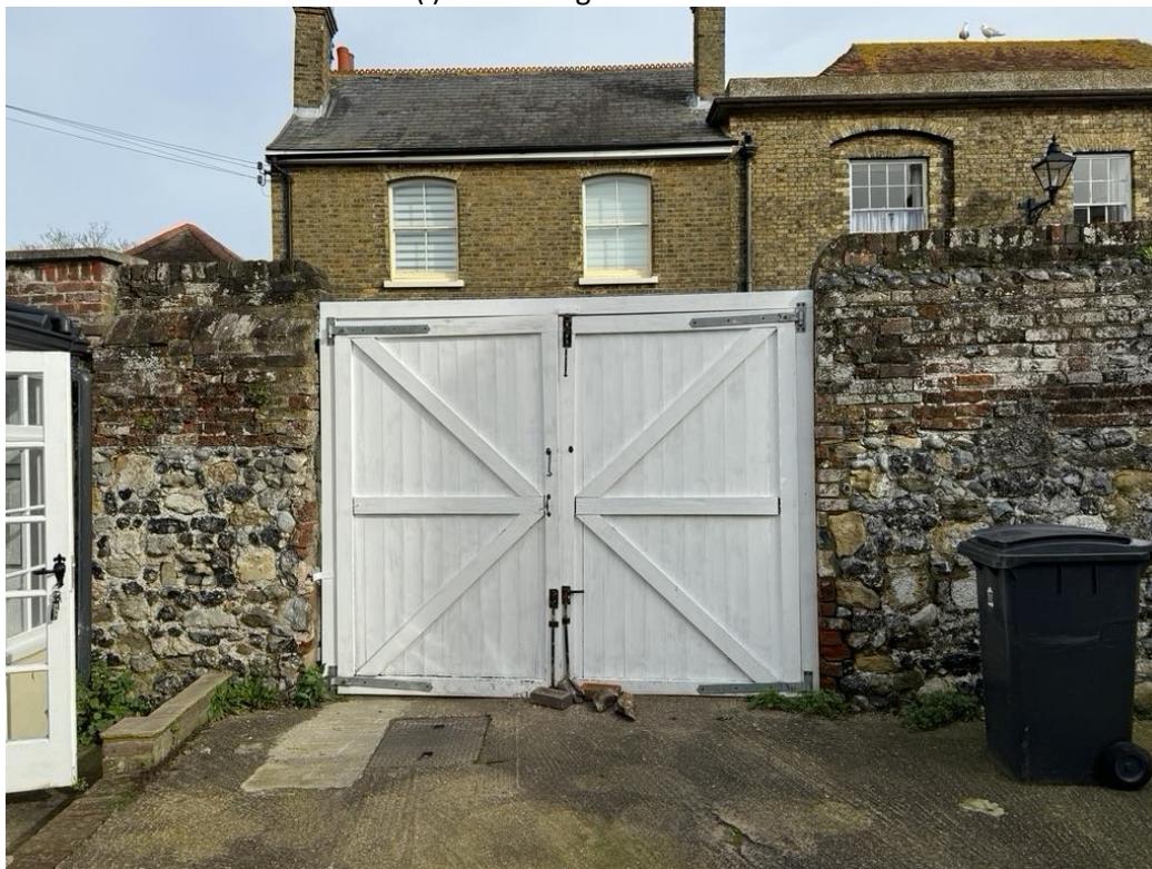
Photo (ii) – view of gates from inside garden courtyard
