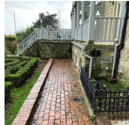
Image 5 – view along eastern elevation of veranda looking south
