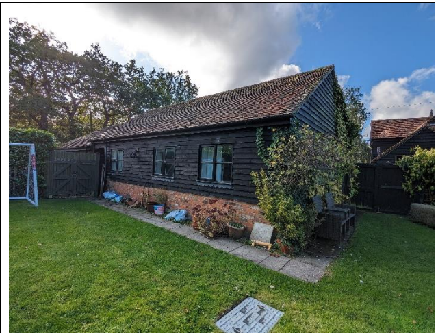
Photograph 2: North and east elevations of the annexe
