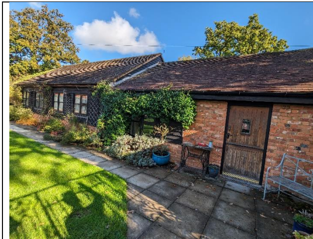
Photograph 1: West elevation of the annexe
