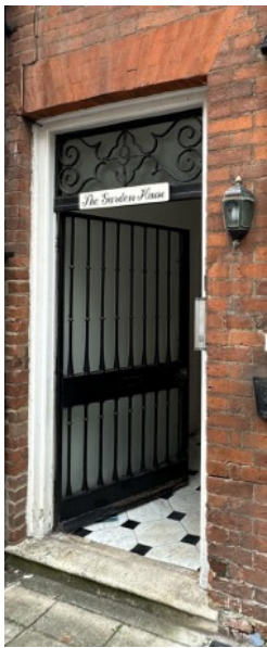
Existing Front Door
