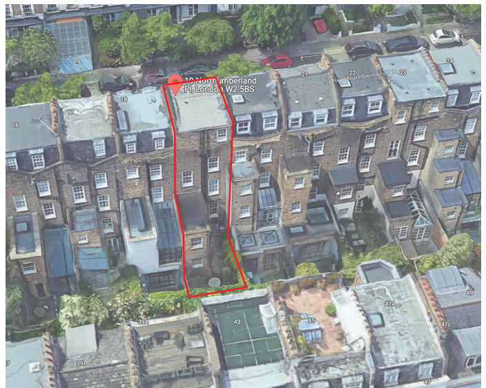
Fig 2.0 Aerial view of rear elevations
