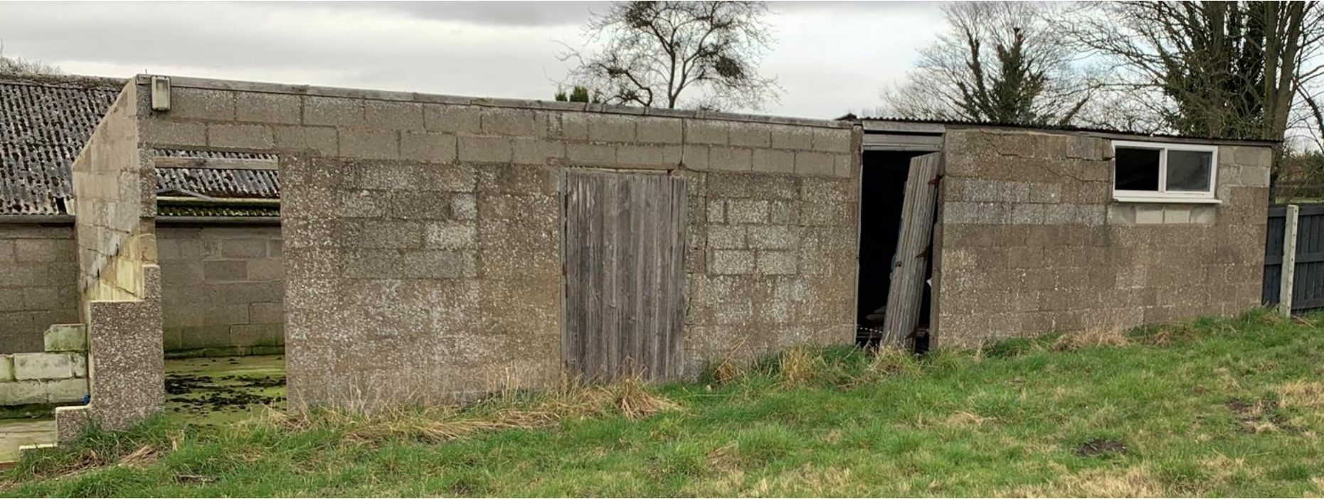
Building to be demolished
