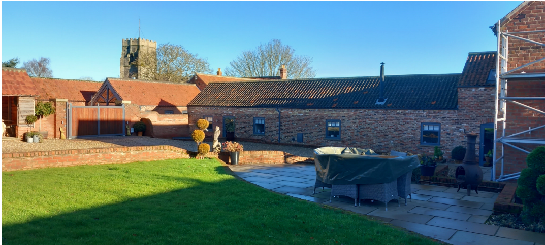
East West elevation of Old Well Barn with adjacent houses behind
