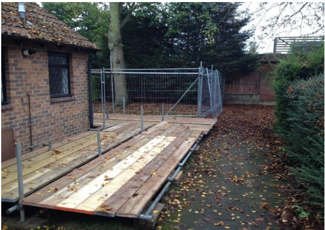
Figure 8 – Specification for scaffold ground protection.
