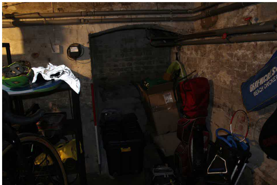
Figure 24 Detail of storage alcove in eastern wall of Room 1. Photograph taken facing east.
