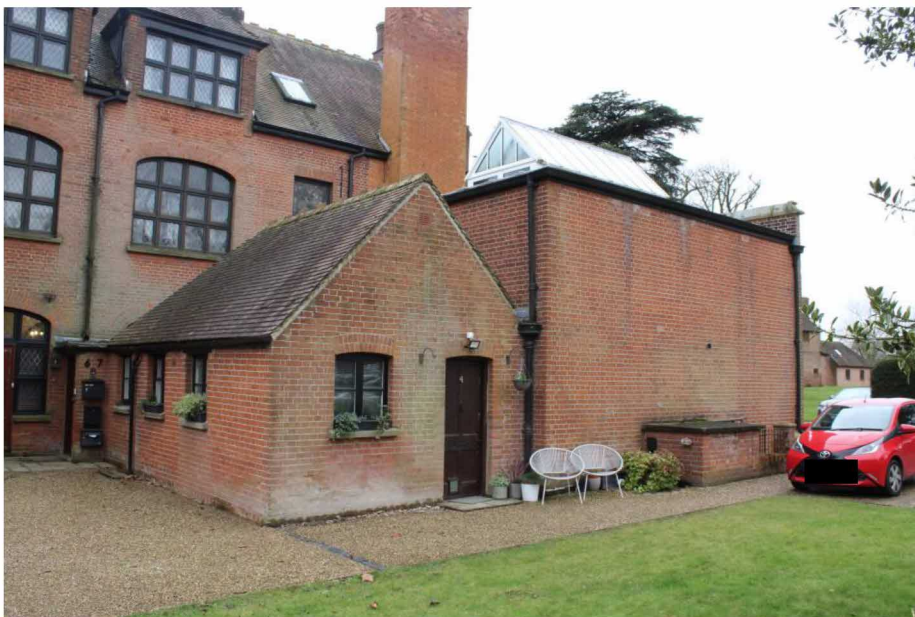
Figure 16 Northern and eastern elevations of 4 Hadham House. Photograph taken facing south-west.
