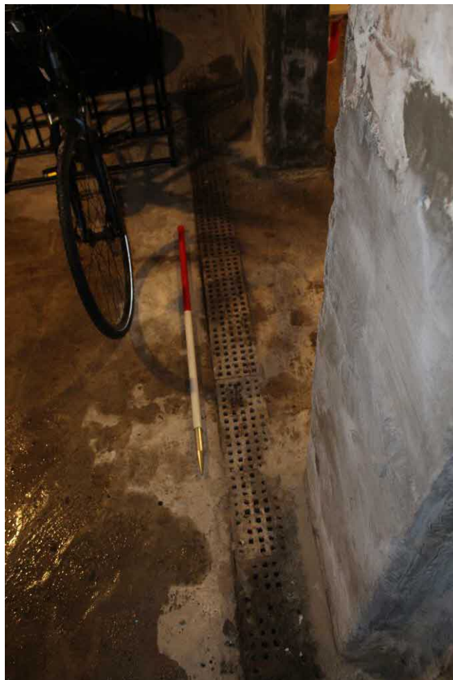
Figure 30 Detail of grated drainage gully in floor of Room 1. Photograph taken facing west.
