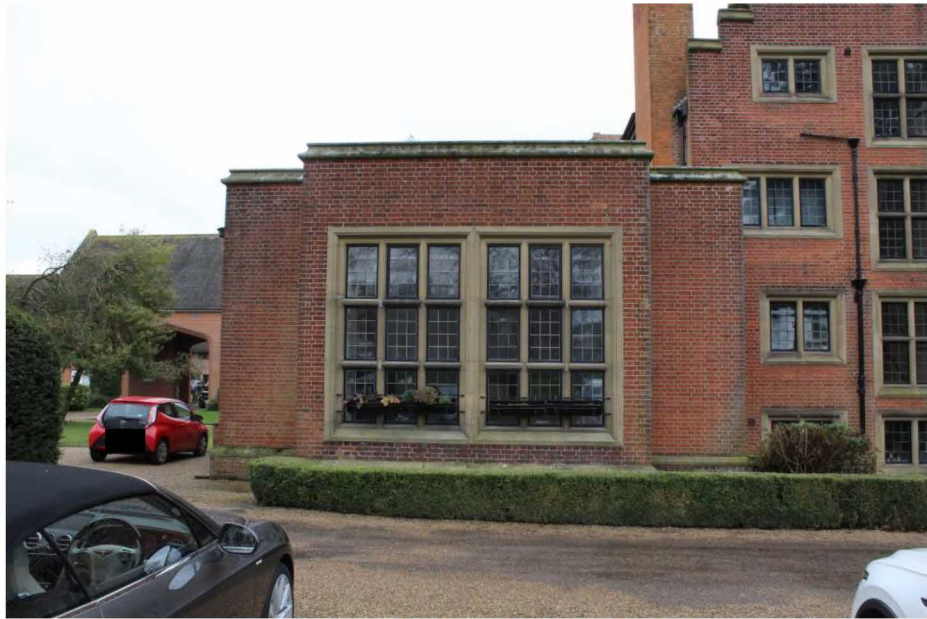
Figure 14 Western elevation of 4 Hadham Hall. Photograph taken facing east.
