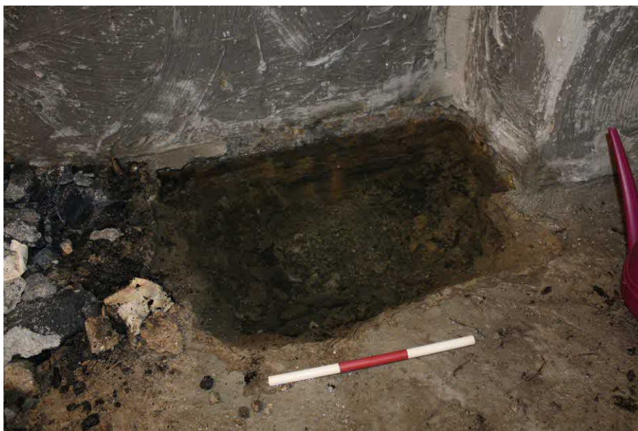
Figure 32 Trial pit excavated in Room 2, showing brick foundations of basement. Photograph taken facing north-east.
