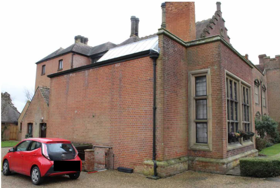
Figure 10 Northern elevation of 4 Hadham Hall, showing access into basement. Photograph taken facing south-east.
