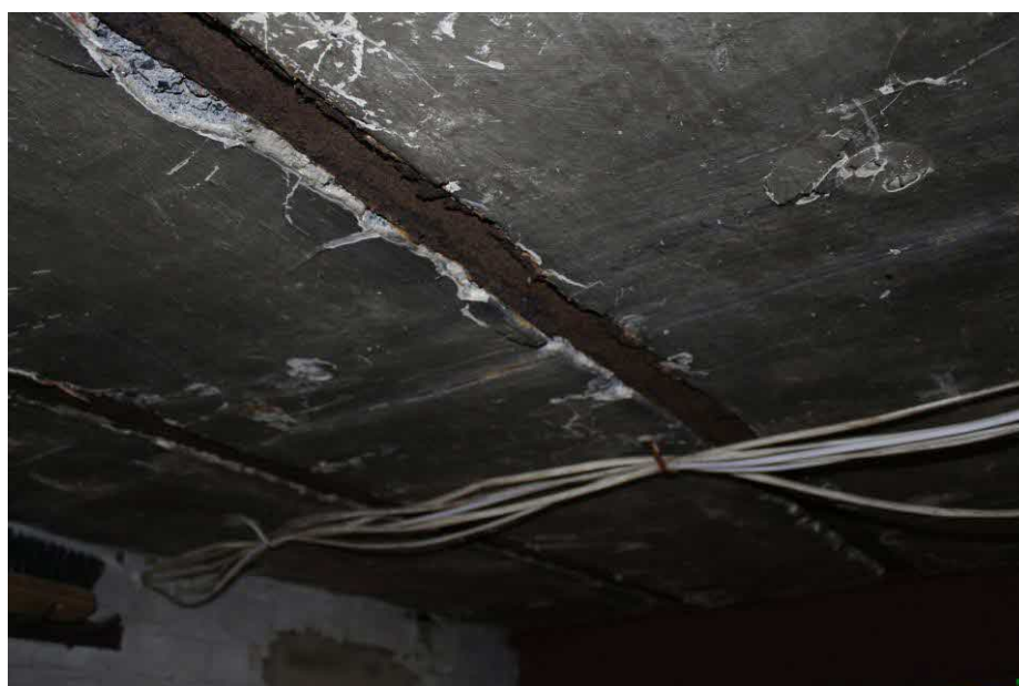
Figure 19 Detail of basement ceiling above Room 1. Photograph taken facing north-east.
