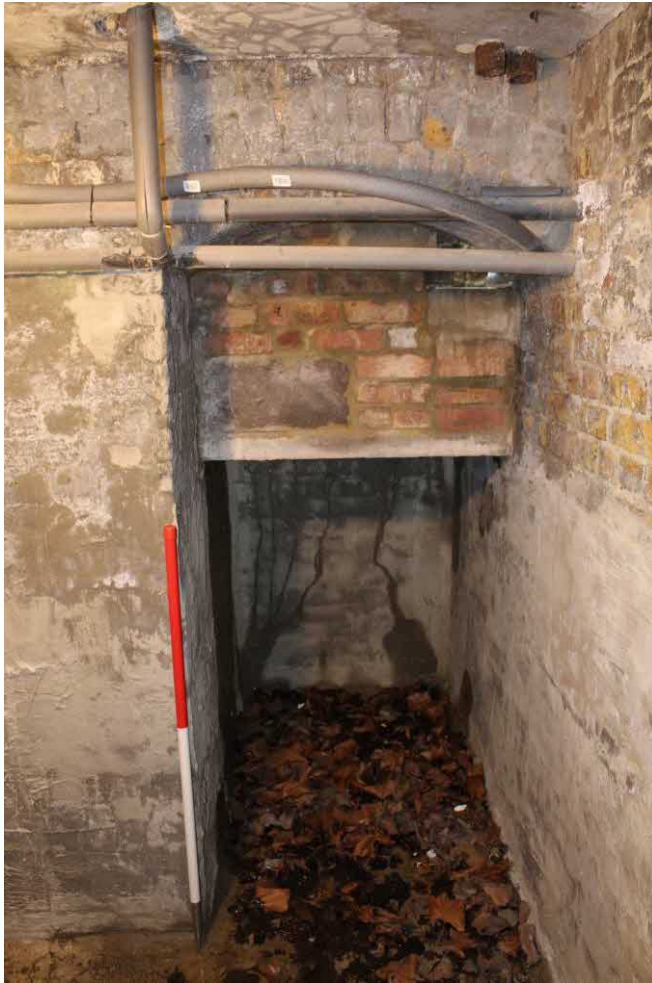
Figure 35 Detail of storage alcove in northern wall of Room 3. Partially blocked by inserted exterior staircase. Photograph taken facing north.
