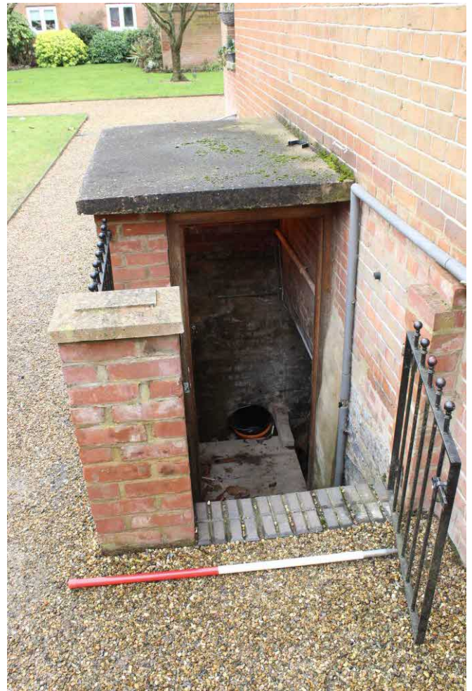
Figure 36 Detail of exterior access into basement. Photograph taken facing east.
