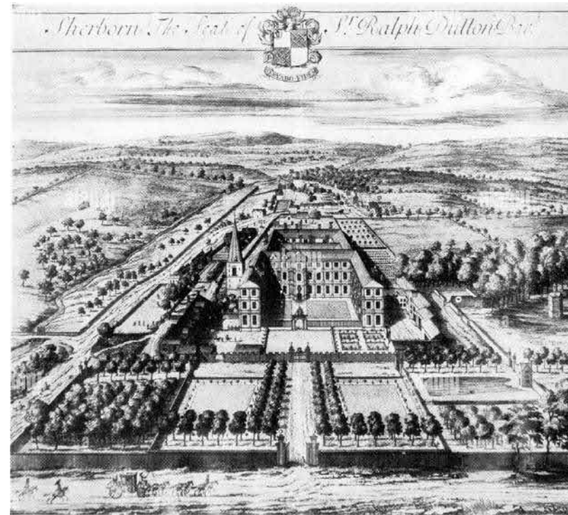
Figure 7: Sherborne House, c.1700, prior to the 19th century rebuilding.
