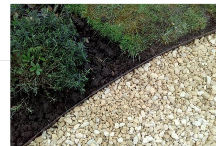
Crushed Cotswold stone driveway with permeable sub-base and steel edging
