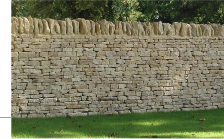
Traditional Cotswold stone boundary wall 1.2m high to follow line of existing pleached trees
