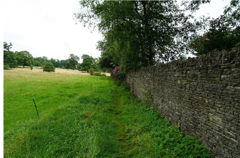
Fig.12 View along footpath 5 of boundary wall to Sherbrook House
