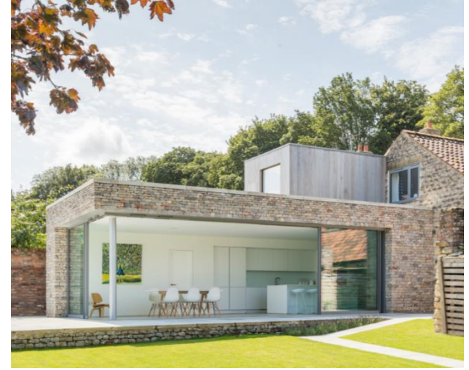
Fig.25 Energy efficient glazing carefully recessed into stonework
