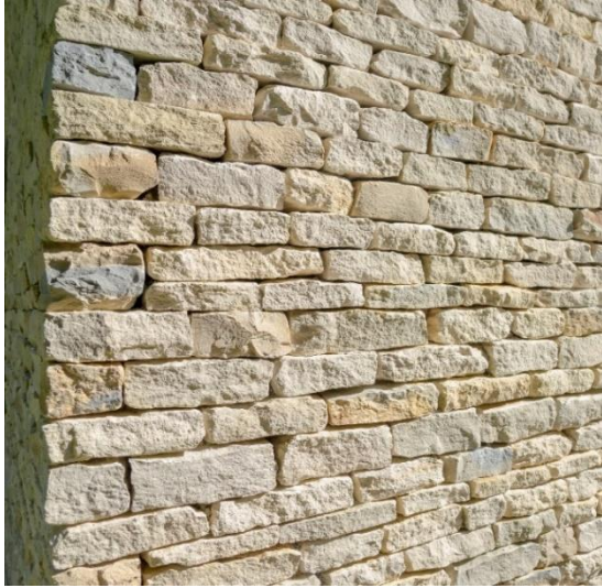
Fig.23 Cotswold Dry-Stone finish using locally sourced limestone and skilled craftsmen
