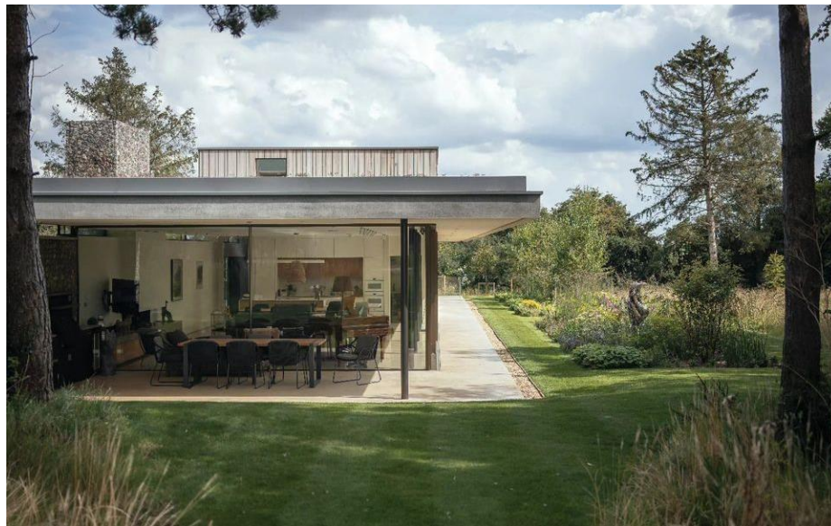
Fig.26 Projecting eaves to accessible modern house with green roof – Arkle Boyce Architects
