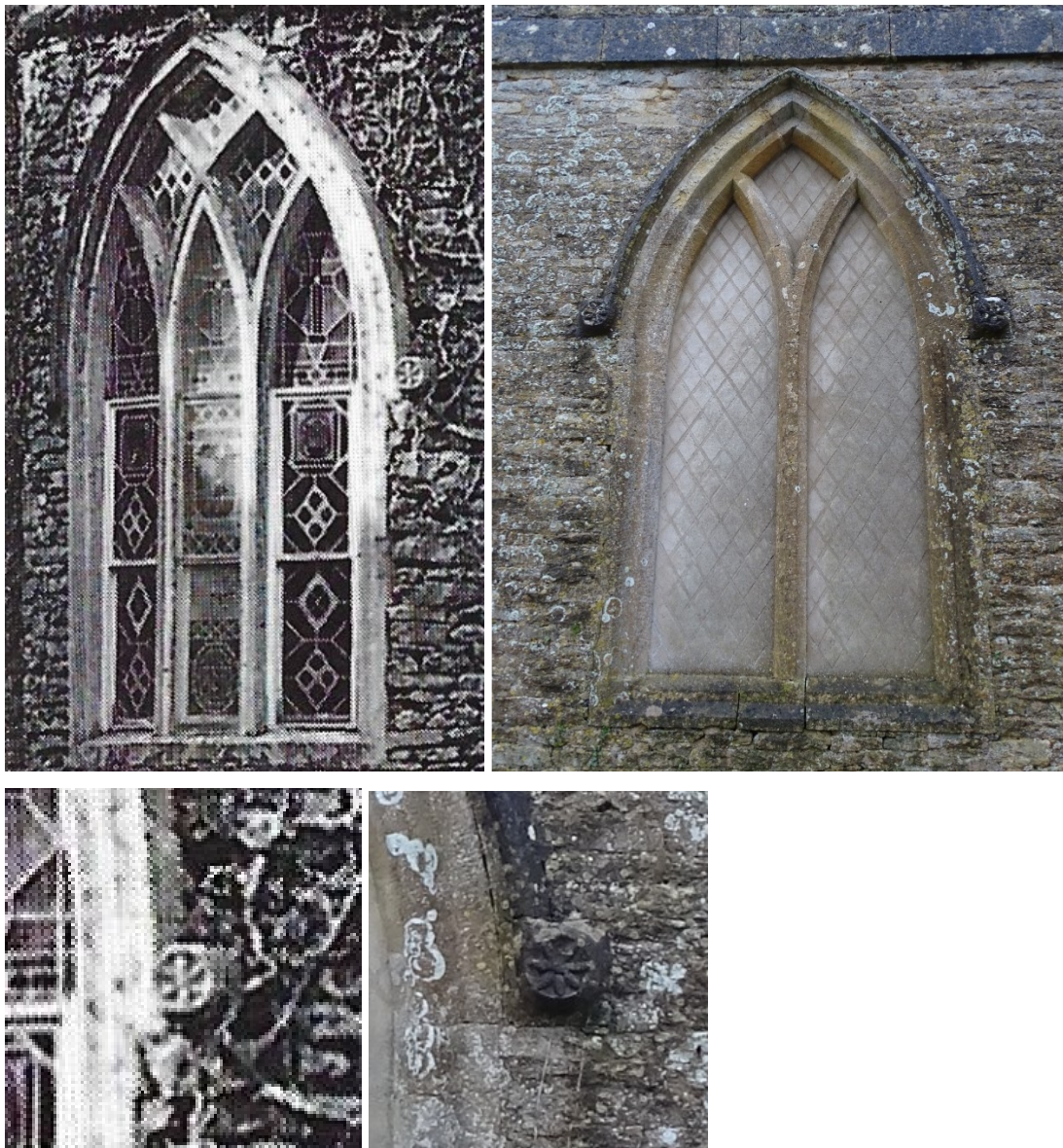
Comparison of the windows in Alfred's Hall (detail from a late nineteenth century photograph) with those on Ivy Lodge. Note the common use of the floral motif on the hood-moulds.
