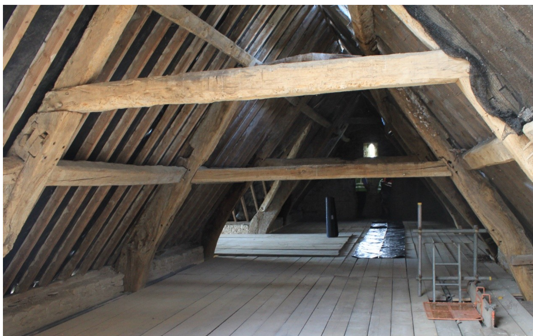
Barn roof timbers, part medieval, during works, artificially lit.
