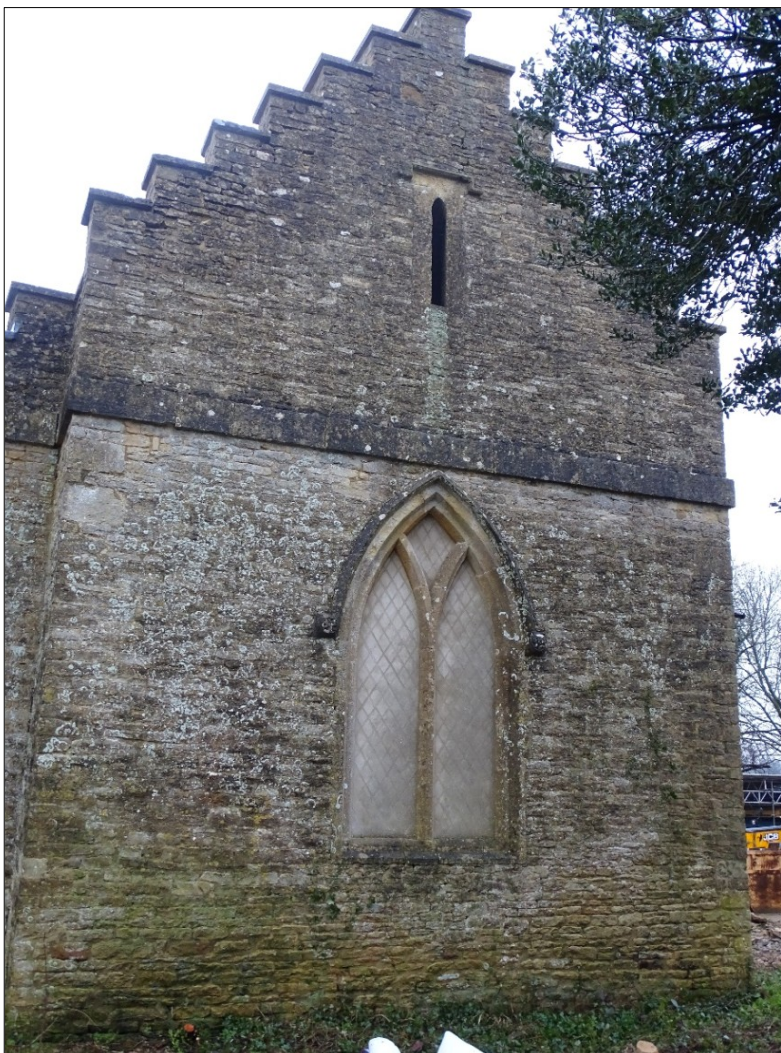
Window 4 of Ivy Lodge, southeast elevation
