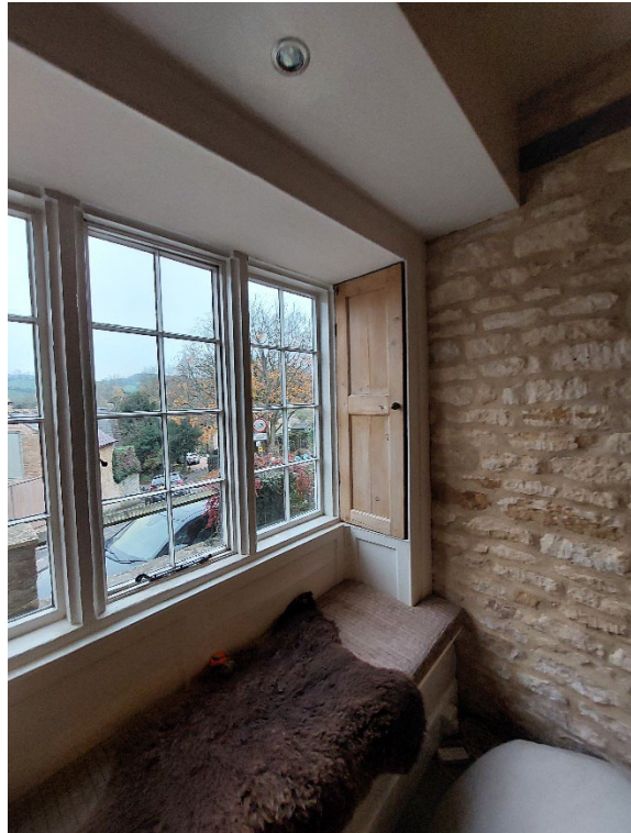
Figure 4.7 – Ground floor Georgian paned window with mullions and panelling, one of several internal historic fenestration surviving.
