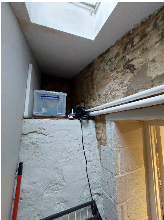
Figure 4.4 – Retaining wall incorporated into modern catslide extension with rooflight.
