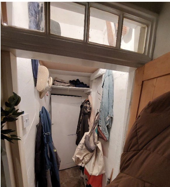
Figure 4.8 – Under stairs cupboard resulting from boxed in staircase. .
