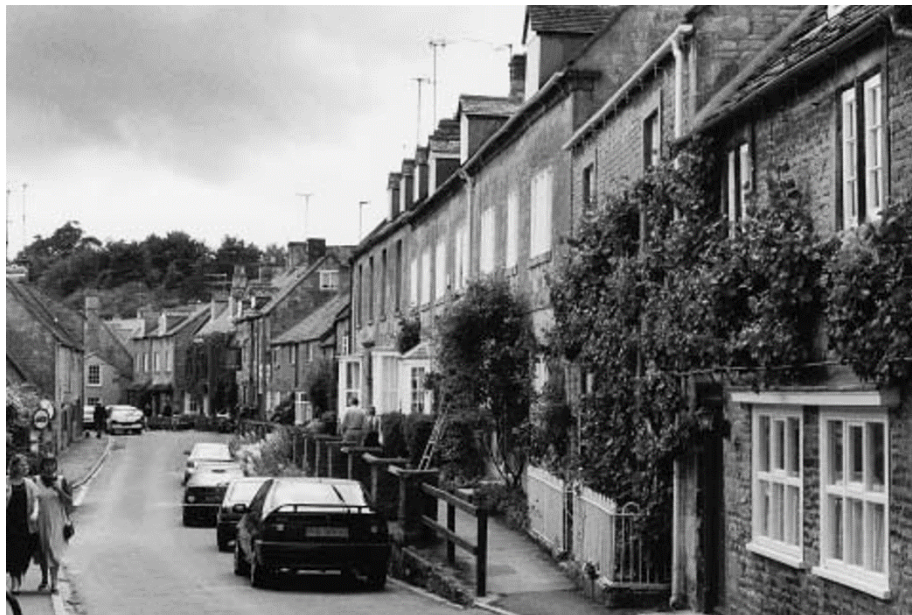
Figure 3.3 – Photo of High Street, Blockley c1950. Source Francis Frith
