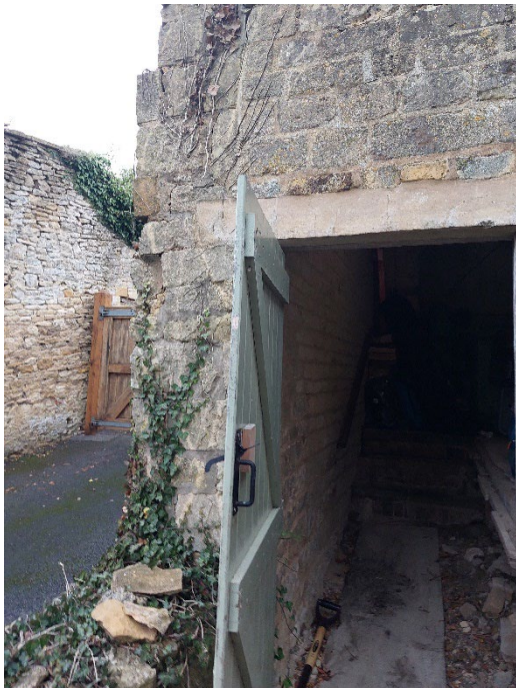
Figure 5.11 – Shows small staircase inside building with elevated timber floor.
