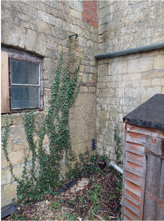
Figure 5.9 – Front elevation of outbuilding.
