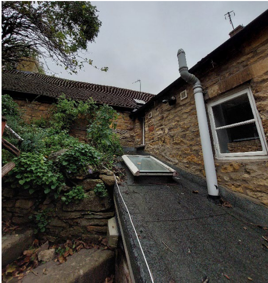
Figure 5.5 Rear extension to Hainault connecting to linear building of The Royal Oak.
