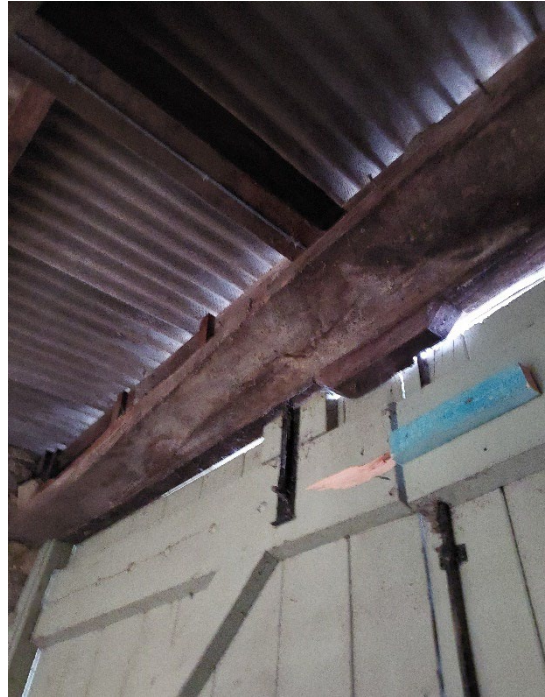
Figure 5.10 – Roof & rear door to outbuilding.
