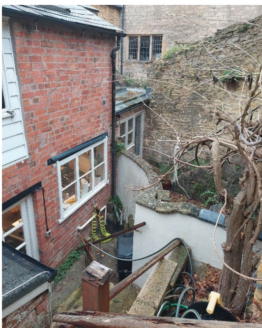
Figure 5.3 - Rear courtyard to Hainault House.
