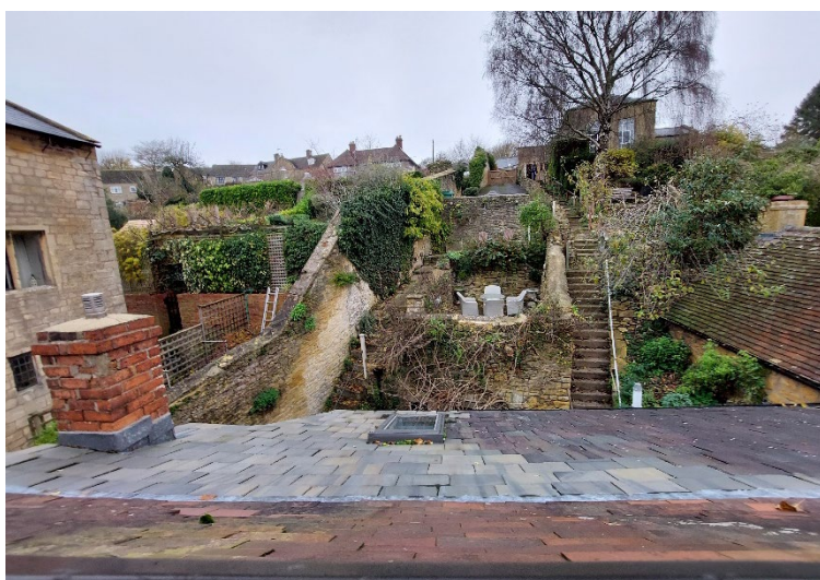
Figure 5.1 – View of first floor catslide roof and rear garden taken from second floor rear window.
