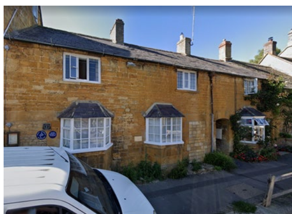
Figure 4.14 – Jasmine Cottage, SW and NE Blocks.
