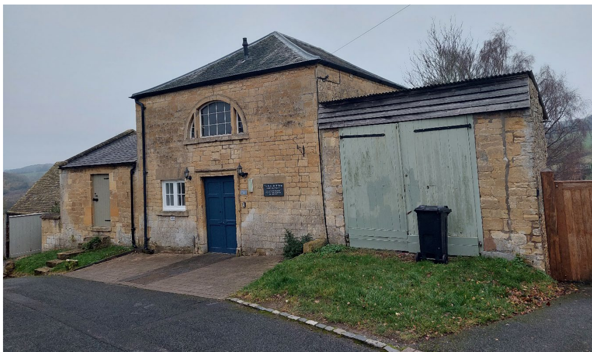
Figure 5.8 – Blockley Village Hall, grade II listed, with Hainault House garage connected (right side of image).
