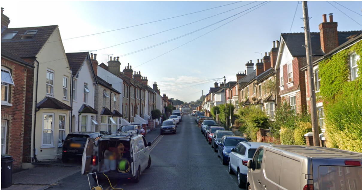
Photo 1. View looking roughly south up Denzil Road. Number 48 is the second house on the left
