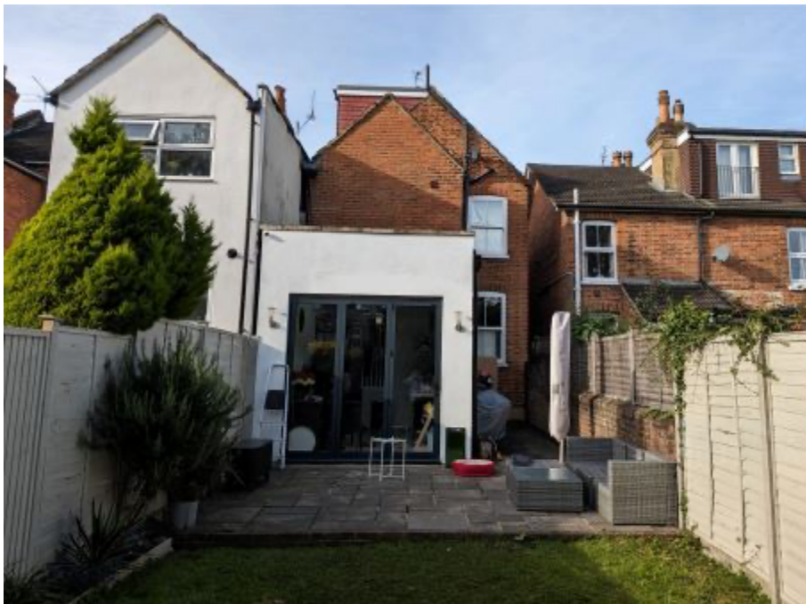
Photo 3. Rear, east, elevation of 48 Denzil Road as existing.
