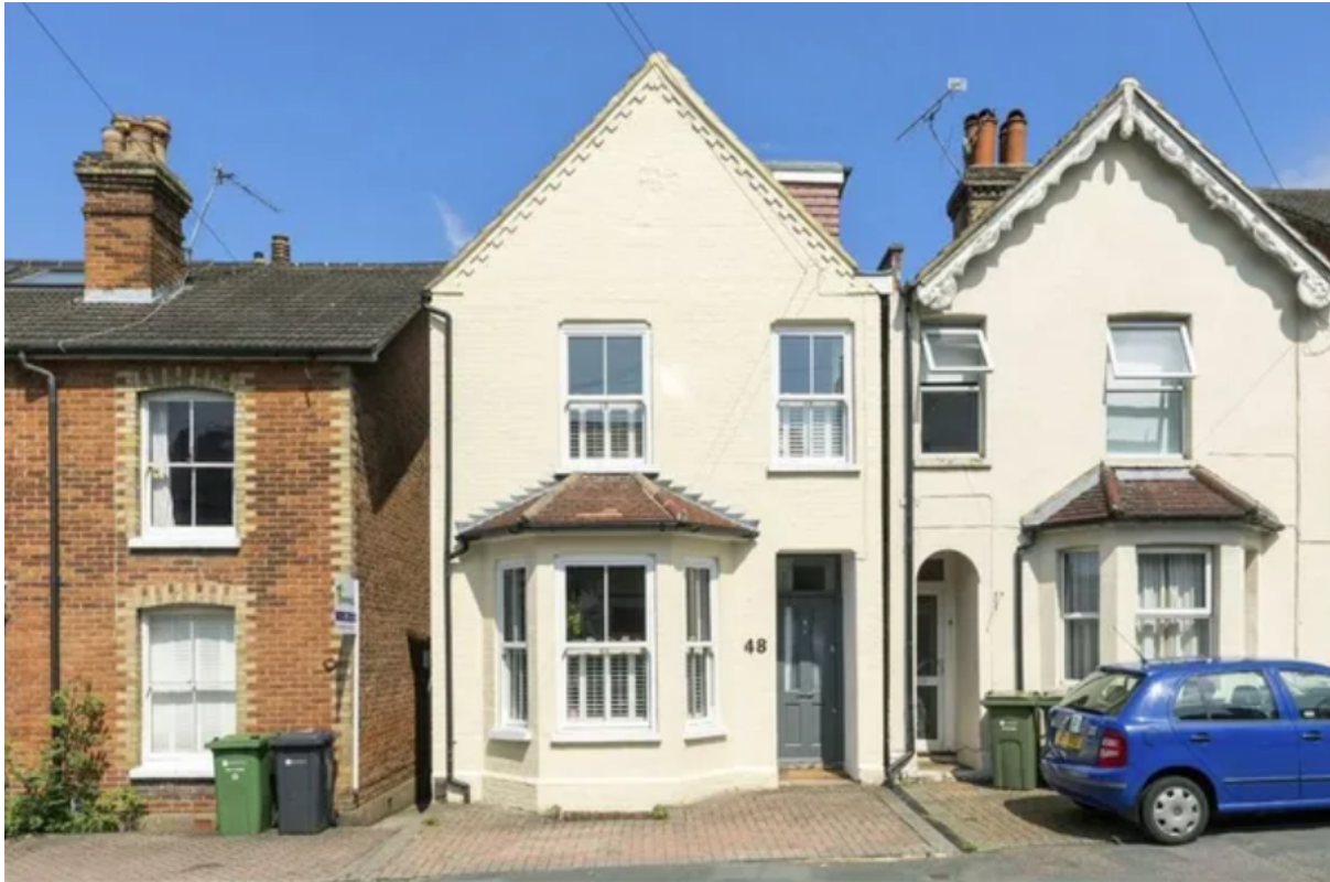
Photo 2. Front, west, elevation of 48 Denzil Road as existing.
